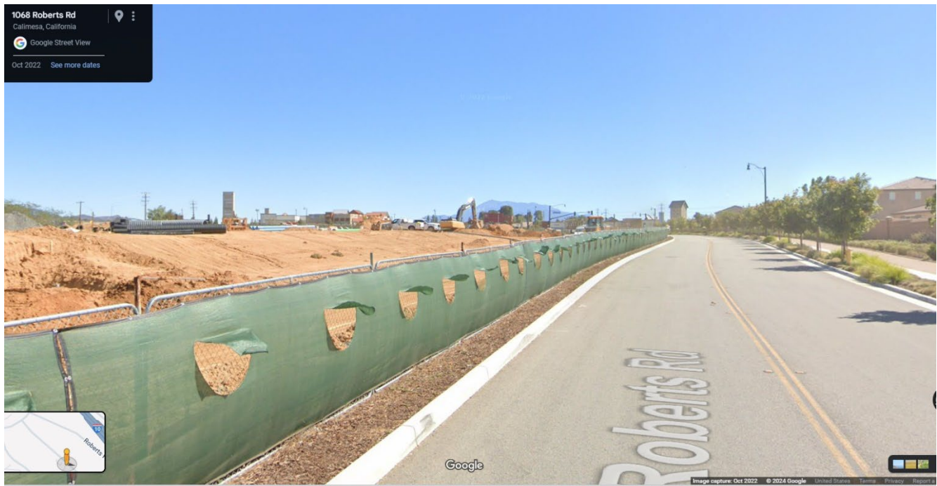
Figure 7 - Cherry Valley indicating development underway - Google Street View 10/2022
