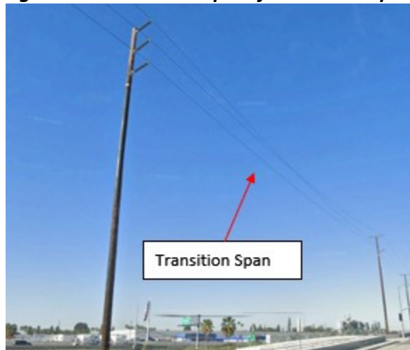
Figure SCE 8-26 - Example of Transition Span
