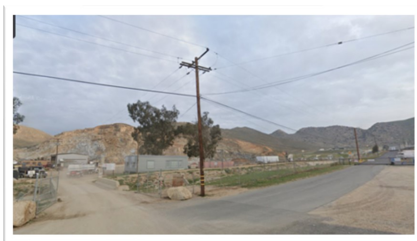
Figure SCE 6-17 - Photo of Location Confirms Need to Convert Designation from Severe Risk to High Consequence
