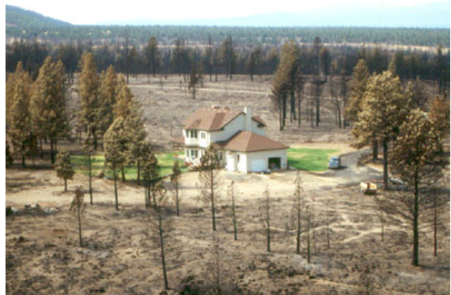
Home surrounded by wildland that survived a fire due to good defensible space.
