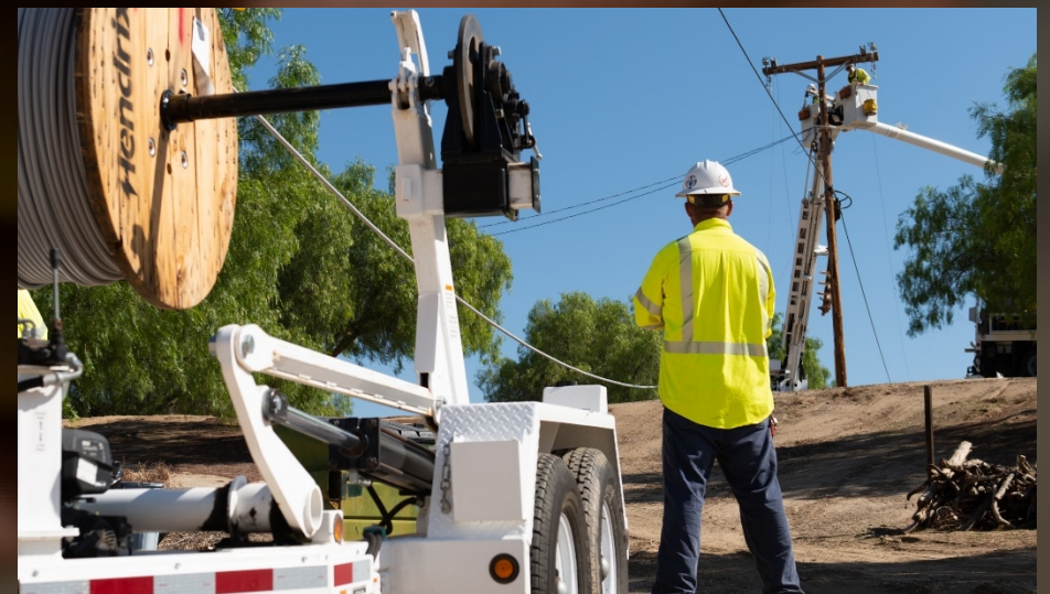
Above photos: SCE crew installing insulated wire
