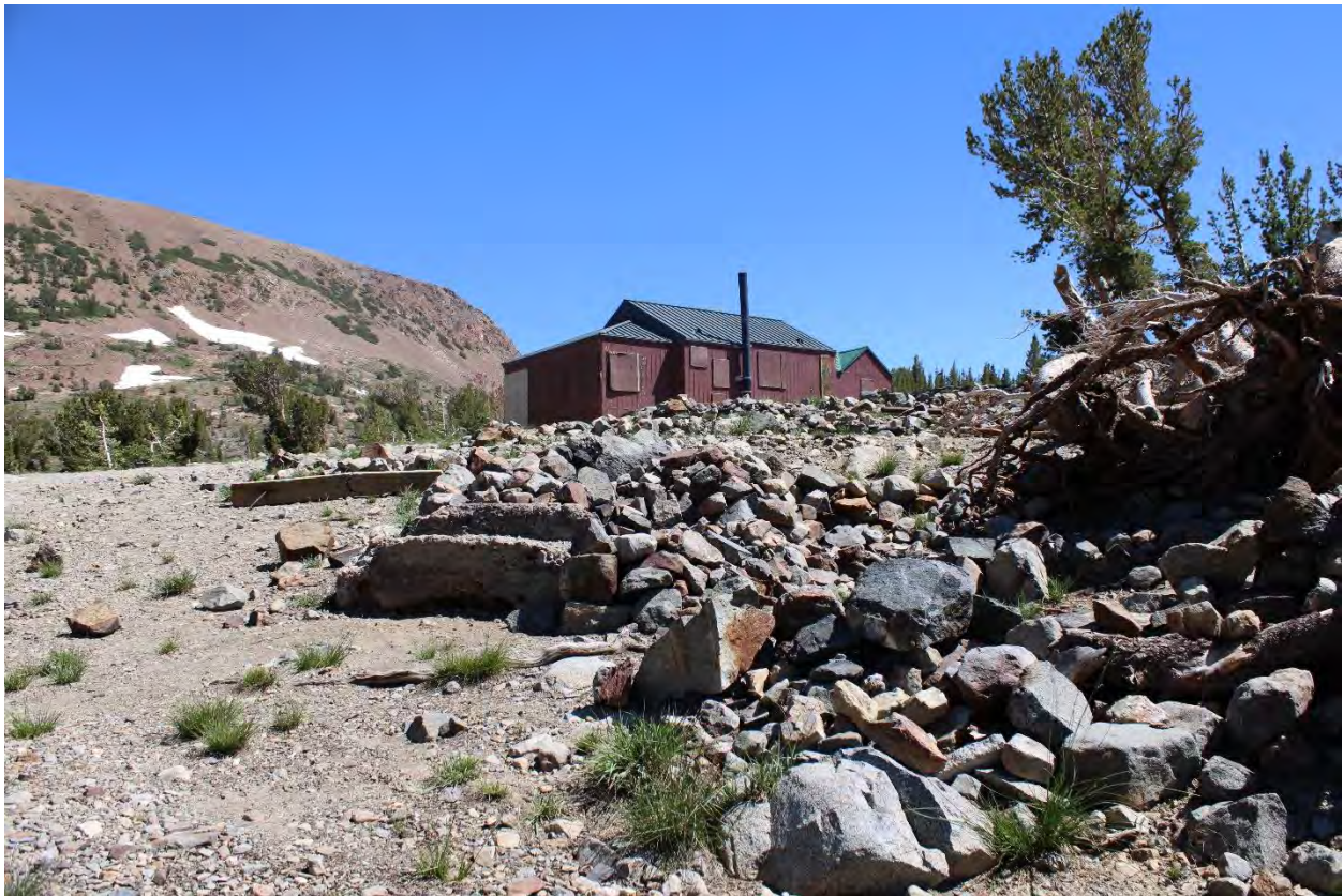
KOP 1, Lower view, looking Southeast
