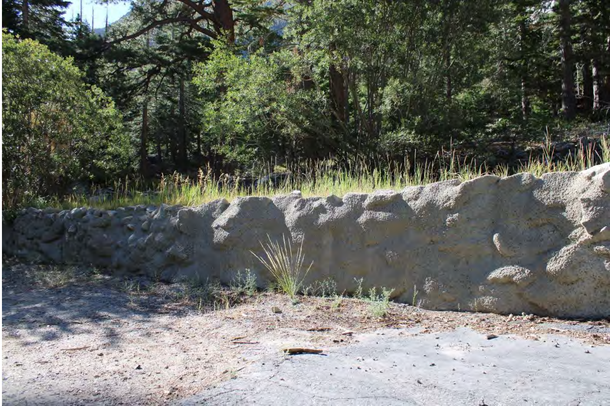
KOP 7, Middle view, looking Southeast
