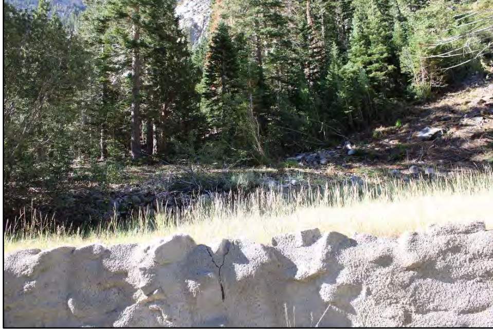
Photo 64. KOP 7 Poole Powerhouse Gate View South.
