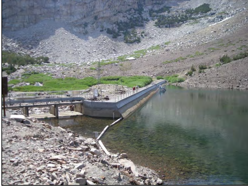
Photo 5. Rhinedollar Dam (Ellery Lake) and Spillway.
