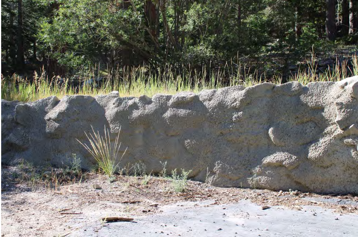
KOP 7, Lower view, looking Southeast
