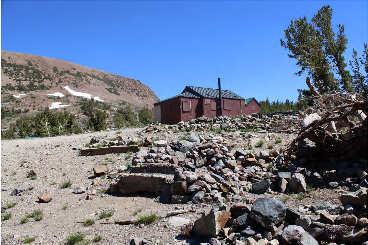
KOP 1, Middle view, looking Southeast
