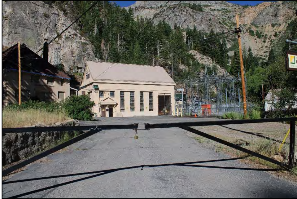
Photo 66. KOP 7 Poole Powerhouse Gate View West.
