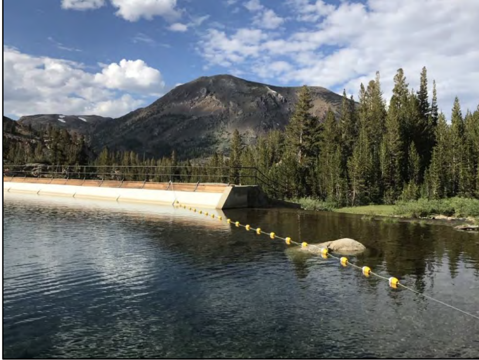
Photo 3. Tioga Dam and Spillway.
