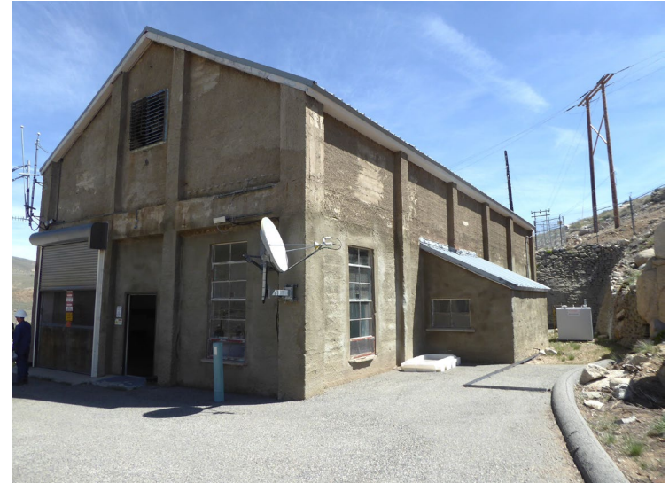
Powerhouse, Lundy Lake Hydroelectric Project, camera facing north, May 2025.
