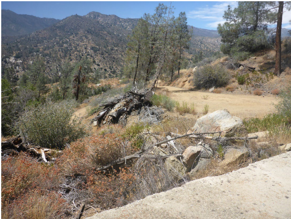
Figure A-26. Overview of Tunnel 10 Spoil Site (view looking downstream from top of exposed tunnel section).
