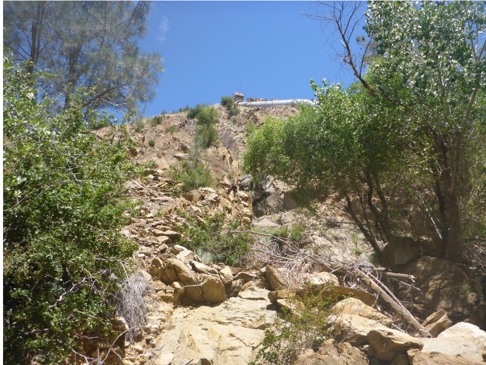
Figure A-55. Cannel Creek Siphon Spillway Channel (view looking upslope).
