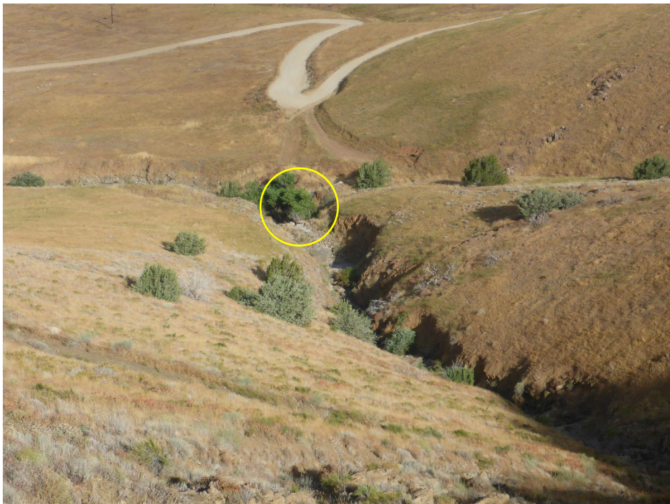
Figure A-60. Top of KR3 Powerhouse Forebay Spillway channel (looking downstream; location of knickpoint in Figure A-59 image indicated by yellow circle).
