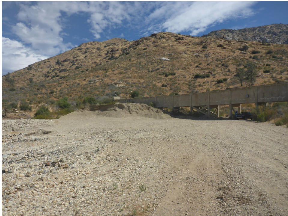
Figure A-42. Spoil material and large pad at Corral North Tunnel 17 Spoil Site. Aggregate stockpile adjacent to exposed tunnel structure in foreground likely imported material for road maintenance.
