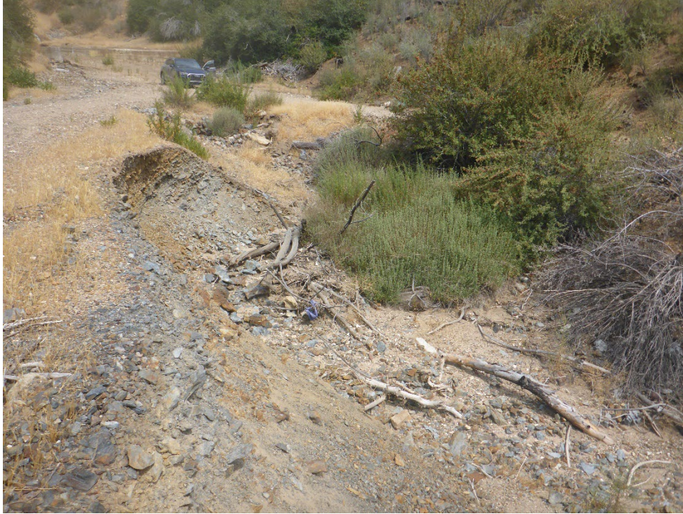
Figure A-51. Semi-active erosion of Tunnel 18/19 Spoil Site along watercourse margin; exposed tunnel section that disrupts surface drainage pattern visible in background behind vehicle (view upstream).
