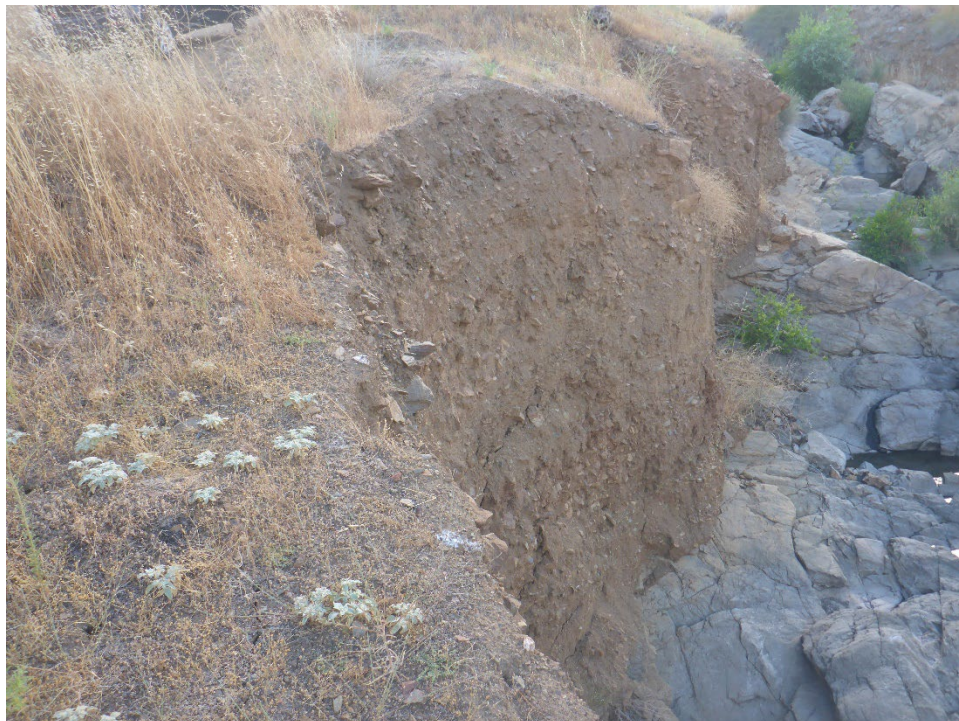
Figure A-56. KR3 Powerhouse Forebay Spillway channel with incision in bedrock and vertical/overhanging banks.
