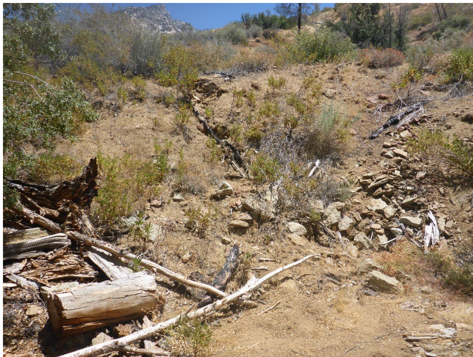
Figure A-28. Small gully formed in road-cut embankment in historical spoil pile at Tunnel 10 Spoil Site; sediment delivered to road surface.
