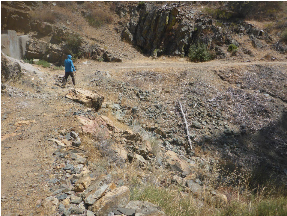
Figure A-40. Spoil material and access road at Tunnel 16/17 Spoil Site with little-to-no active erosion.
