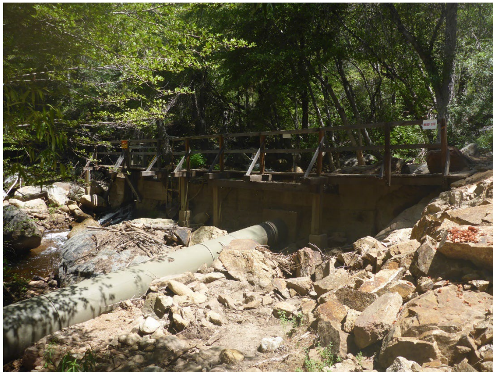
Figure A-18. Downstream side of Salmon Creek Diversion Dam with coarse colluvium from minor rockfall erosion along Left (south) channel margin (view looking upstream).
