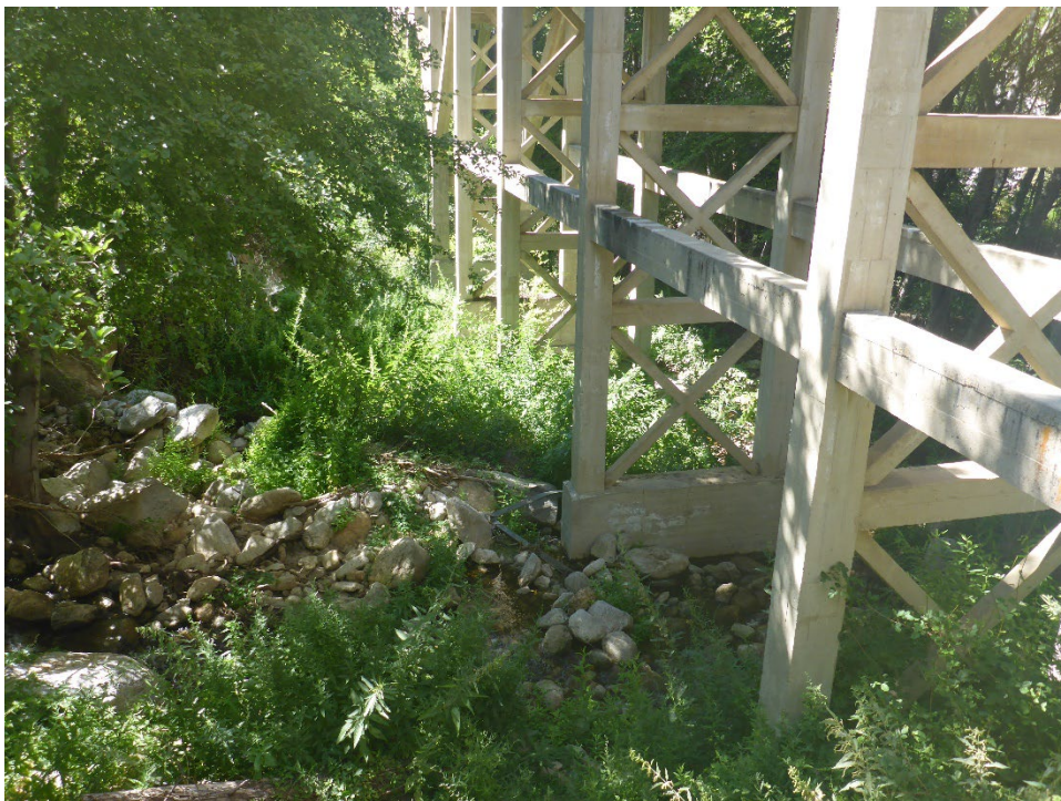
Figure A-44. Concrete footings of elevated flume with minor erosion and sedimentation at Corral Creek crossing.
