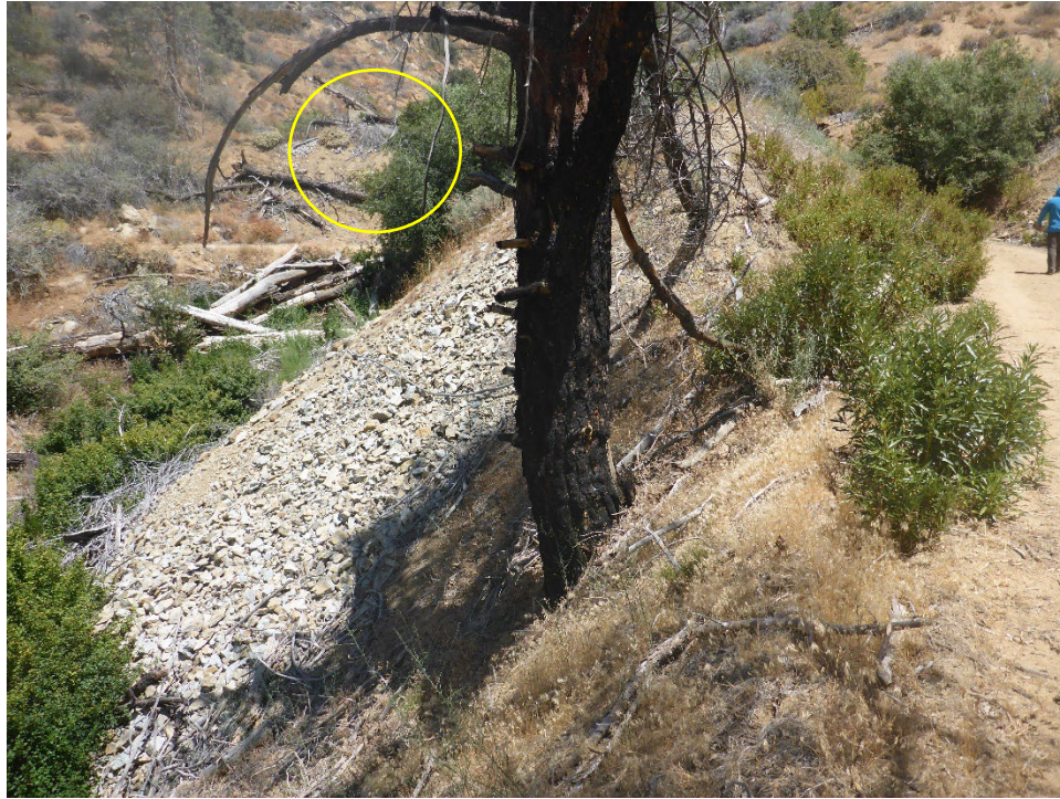
Figure A-27. Access road cut through historical coarse spoil pile material at Tunnel 10 Spoil Site (view looking upstream from left bank [south side]). Small section of exposed tunnel visible (circled in yellow), near location of Figure A-26 Image.
