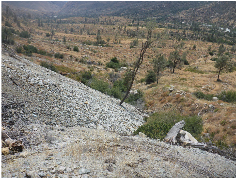
Figure A-32 Outer edge of Tunnel 12/13 Spoil Site with little-to-no active erosion (view looking downslope with Kern River in foreground).
