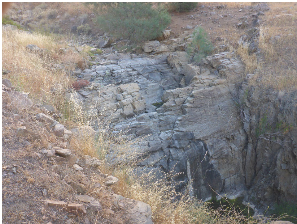
Figure A-58. Knickpoint in KR3 Powerhouse Forebay Spillway channel; few loose or separated blocks in knickpoint face indicate relatively stable feature.
