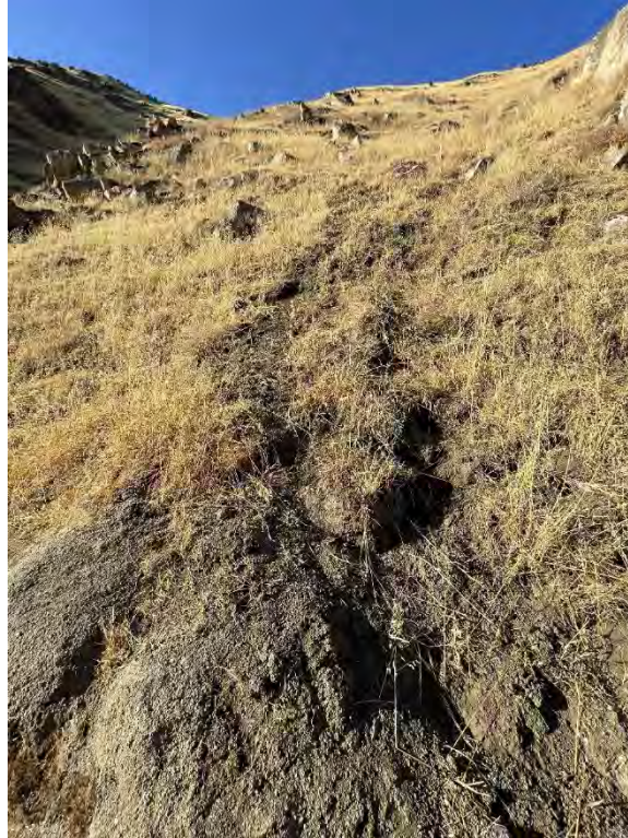
Photo D-1. August 27, 2024. Adit 17 & 18 Trail. Example of hillslope erosion present within steep, grassy trails.
