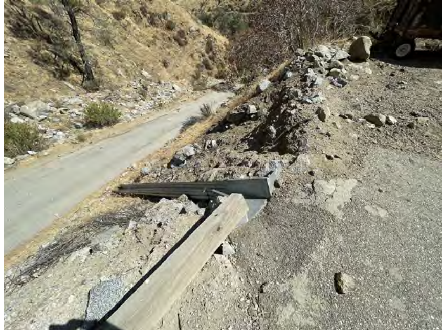
Photo D-15. August 26, 2024. Stark Creek Road. Example of steel slope drain in good condition, which are present throughout Stark Creek Road.
