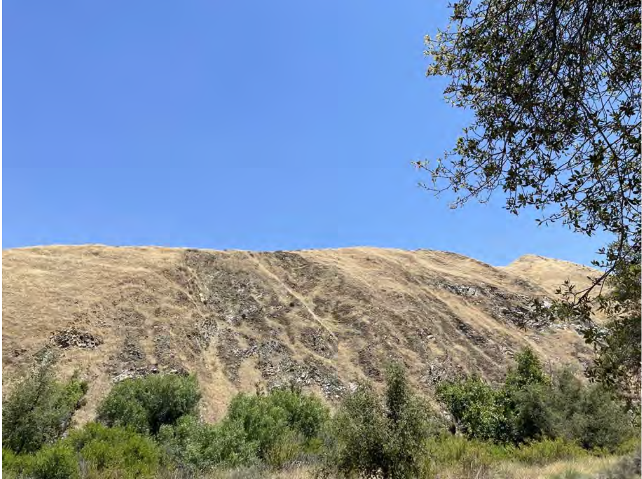
Photo A-14. Rilling/Landslide RB-1
