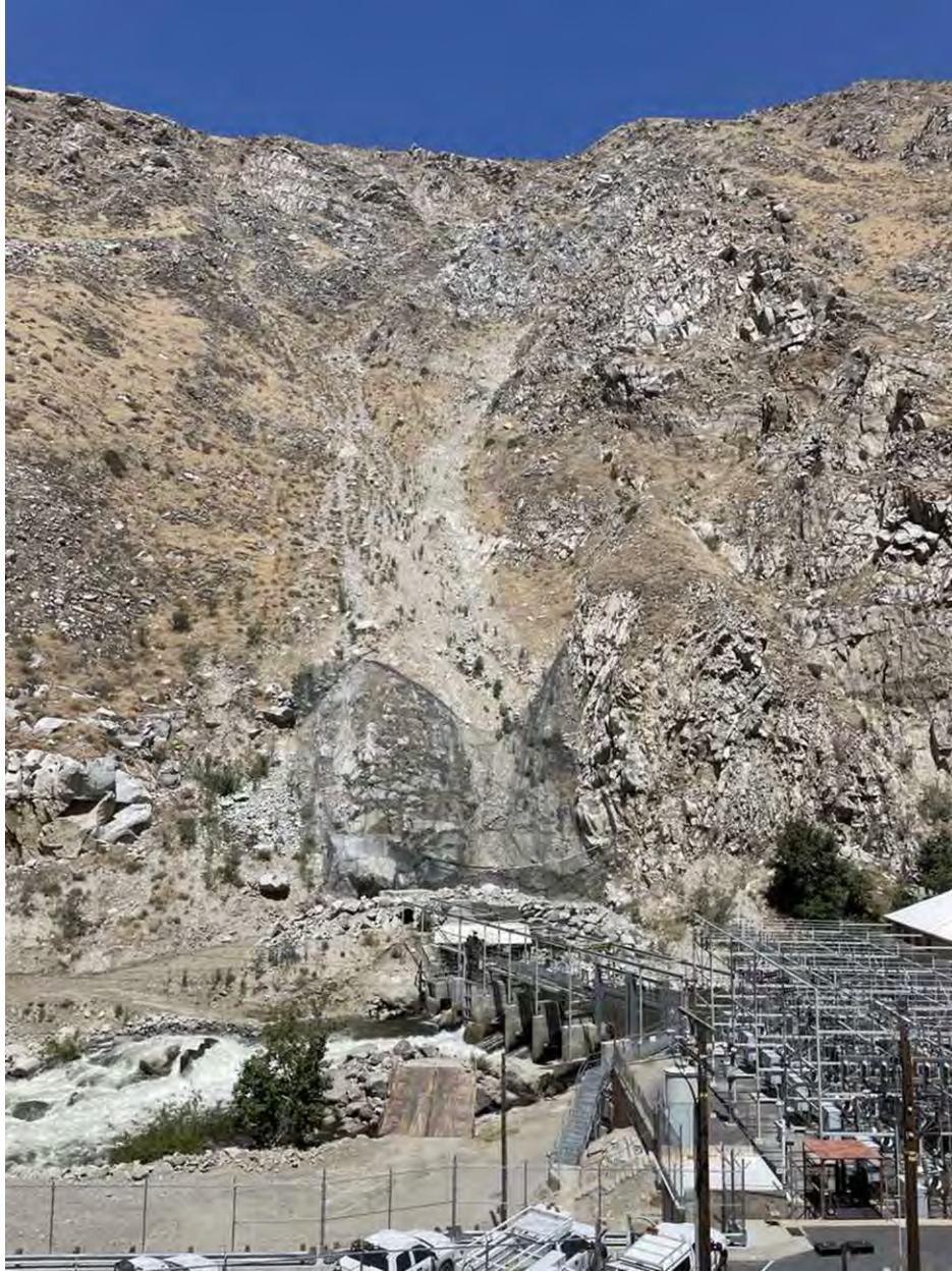
Photo A-17. Natural Rockslide at KR1 Powerhouse
