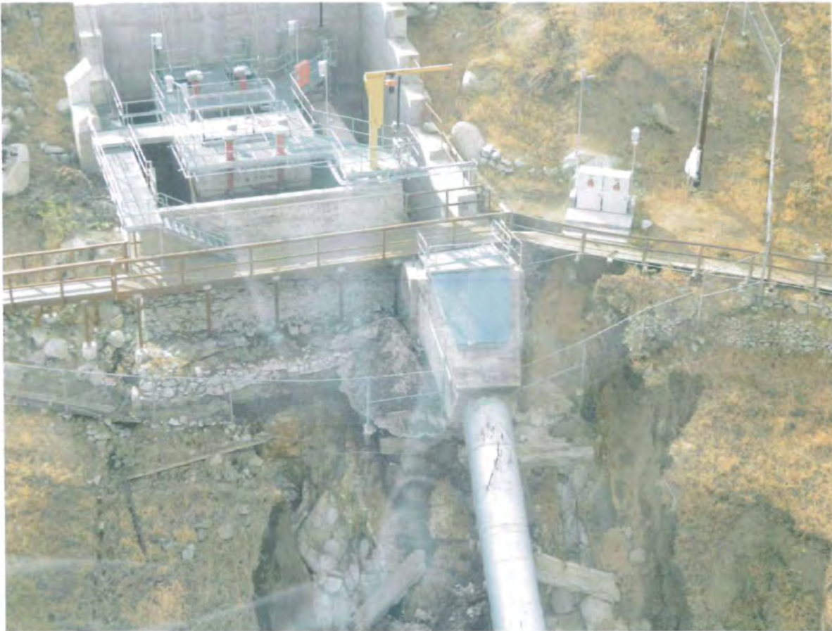
Kern River No. 1 Forebay
