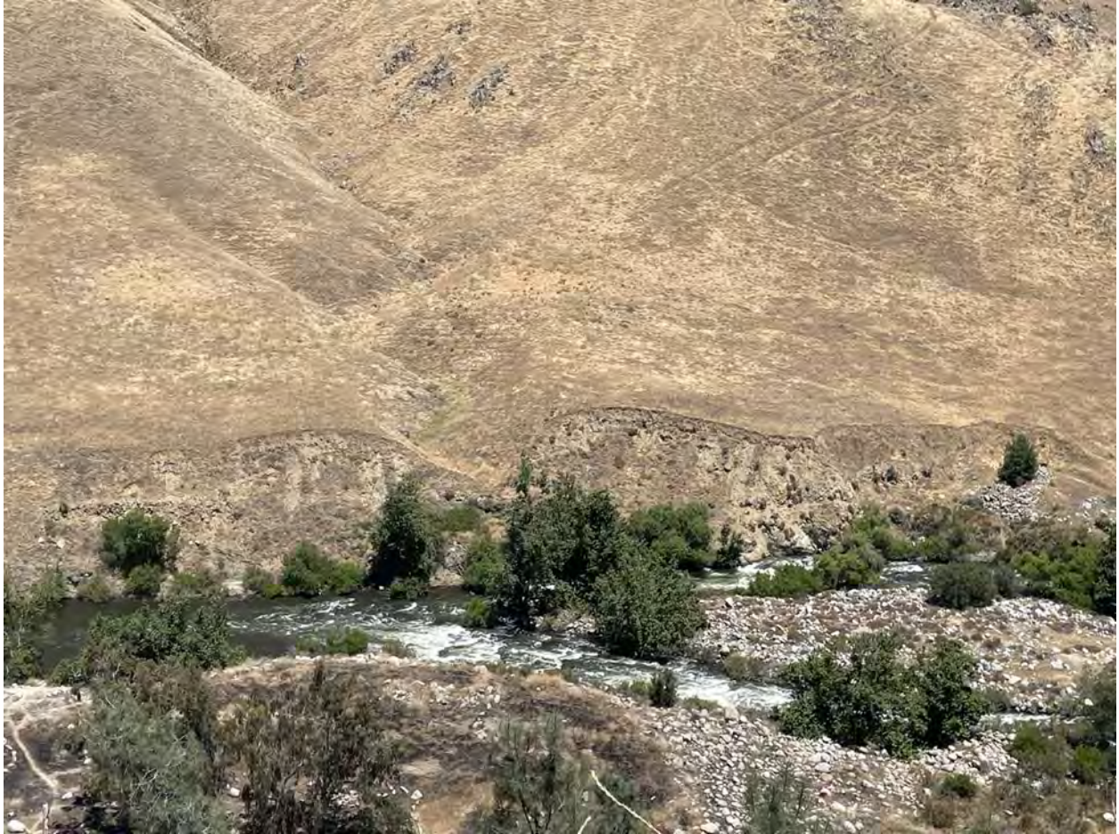
Photo A-10. Bank Erosion RB_1
