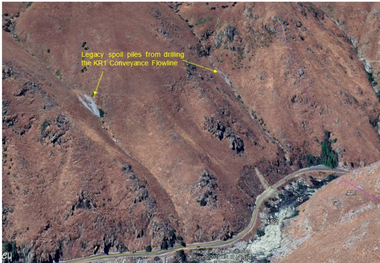
Figure 5-1. Example of Legacy Spoil Piles from Drilling the KR1 Conveyance Flowline.
