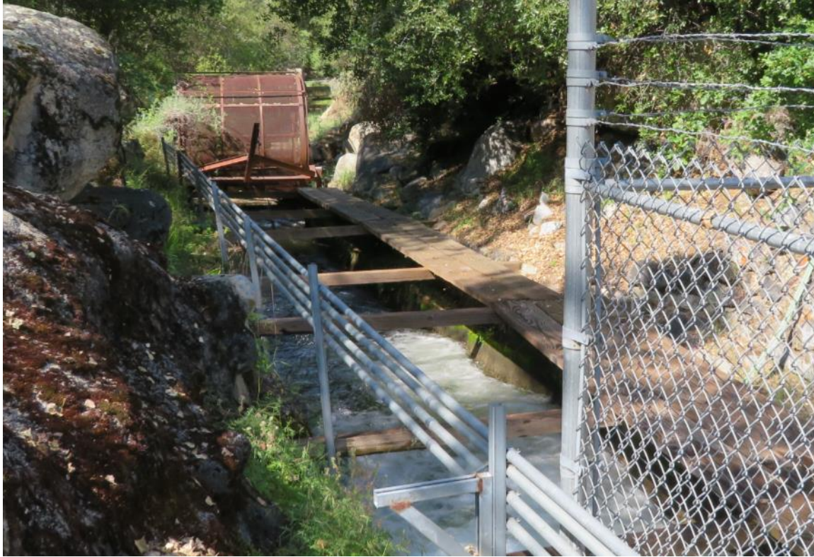
Figure AQ 9-9. Kaweah No. 2 Flowline Fishwheel.
