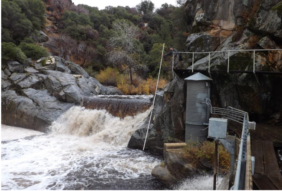
Figure C-5. Image of project barrier at Kaweah No. 1 Diversion Dam. Staff with stadia rod on left bank for scale.
