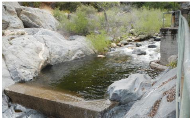
Figure AQ 9-2. The Kaweah No. 1 Flowline Intake, immediately upstream of the Kaweah No. 1 Diversion (top – intake trash screen; bottom left – diversion dam; bottom right – looking down on intake and slide gate gear).
