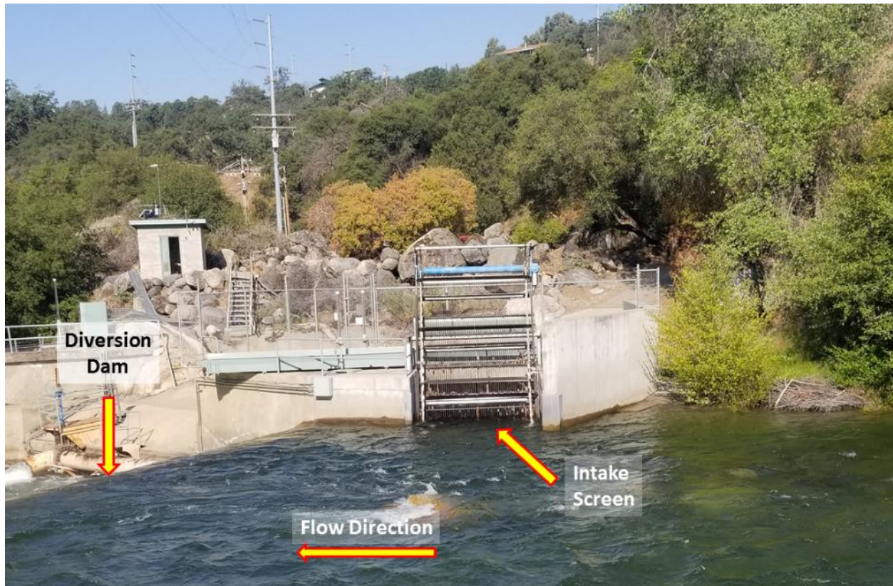
Figure AQ 9-7. The Kaweah No. 2 Flowline Intake, immediately upstream of the Kaweah No. 2 Diversion Dam. Flow is from right to left in the image.
