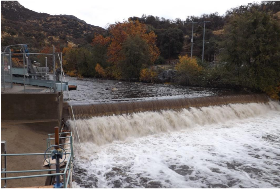
Figure C-2. Image of project barrier at Kaweah No. 2 Diversion Dam. Staff holding stadia rod on left side of image for scale.
