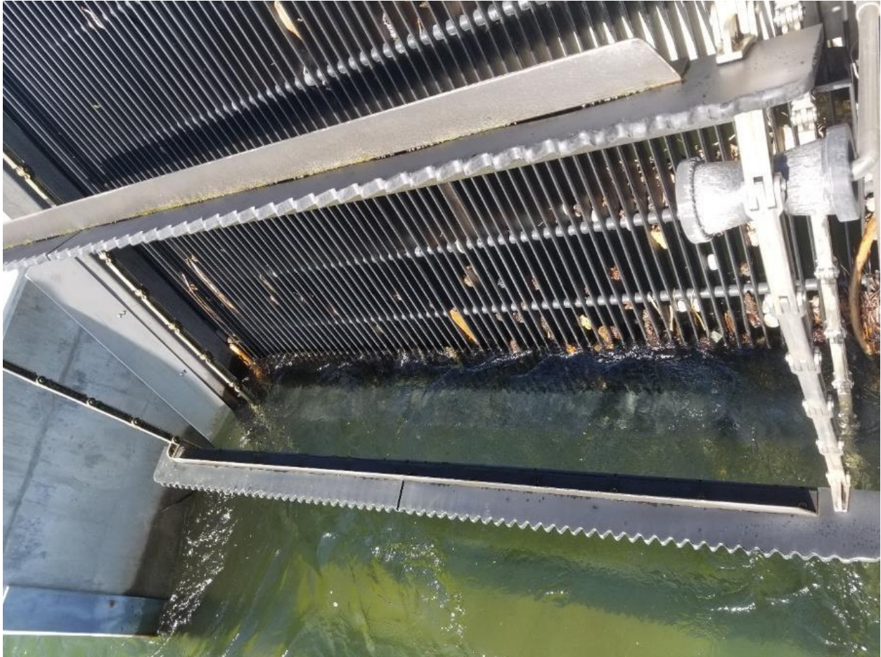
Figure AQ 9-8. Detail, looking down on the Kaweah No. 2 Flowline Intake Grate. Flow is from right to left in the image.
