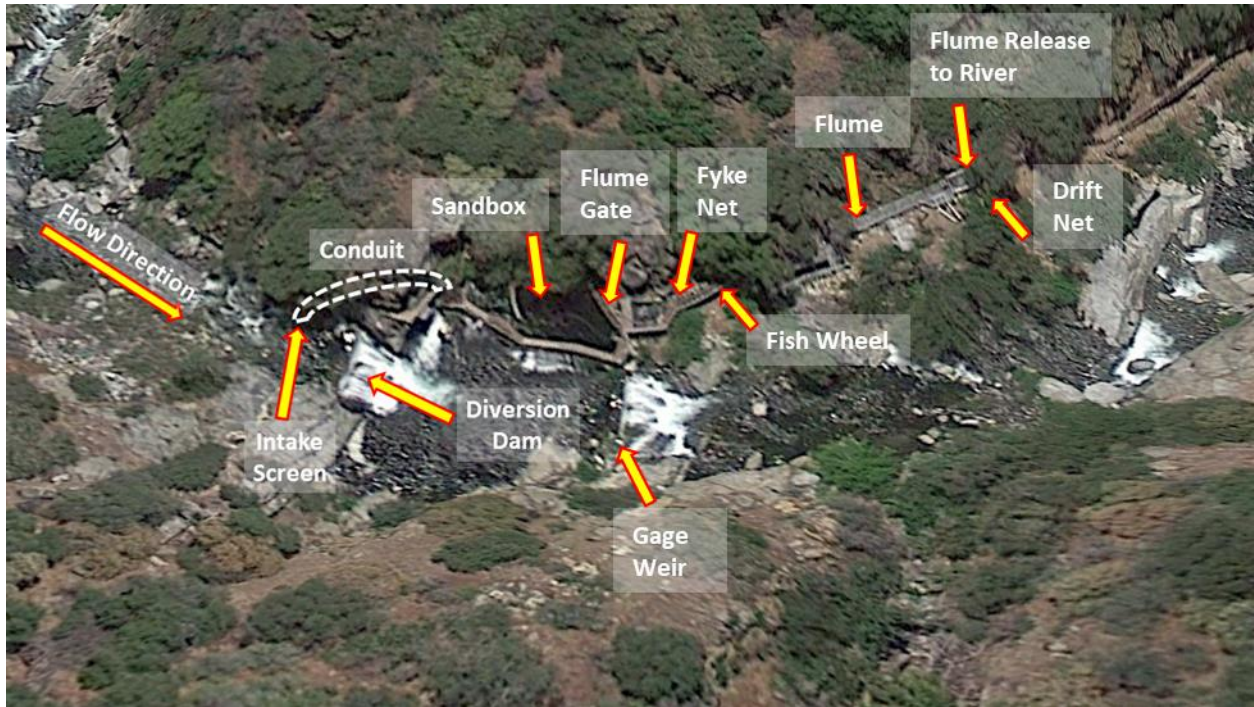
Figure AQ 9-1. Aerial view of the Kaweah No. 1 Flowline Intake with key features labeled.
