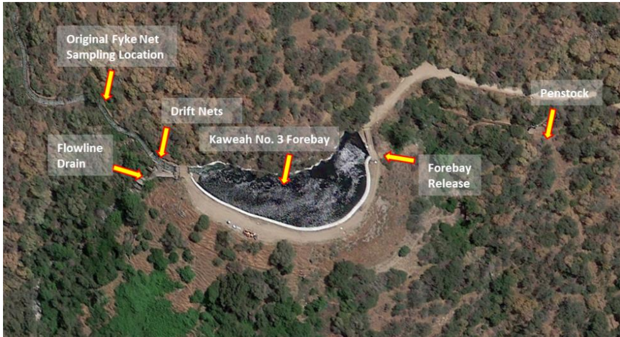
Figure AQ 9-11. Aerial view of the Kaweah No. 3 Flowline, Forebay, Drains, and Penstock.
