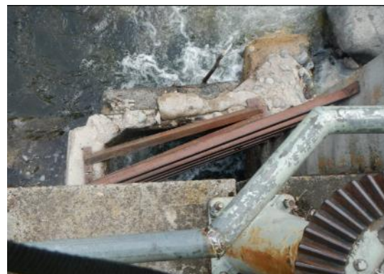
Figure AQ 9-2. The Kaweah No. 1 Flowline Intake, immediately upstream of the Kaweah No. 1 Diversion (top – intake trash screen; bottom left – diversion dam; bottom right – looking down on intake and slide gate gear).
