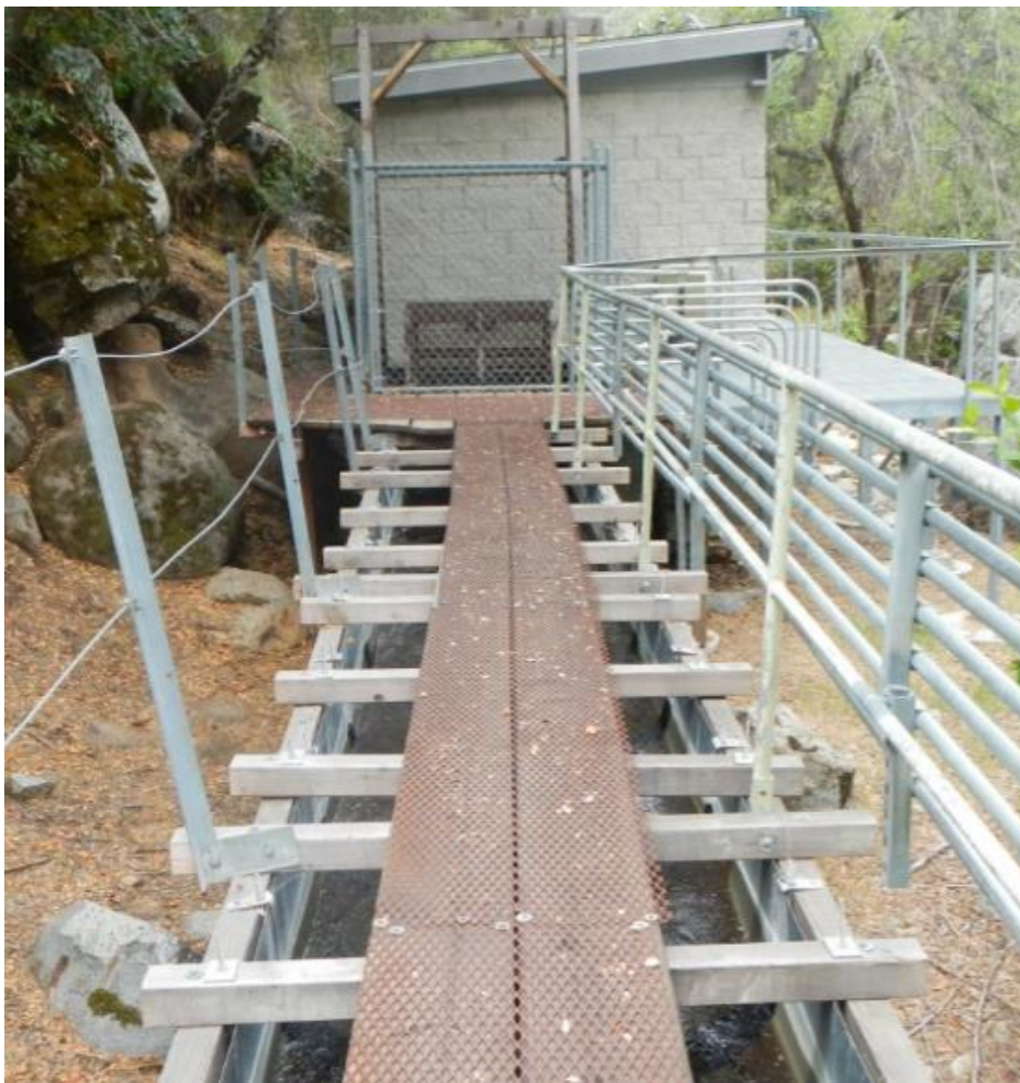
Figure AQ 9-4. Kaweah No. 1 Flowline Fishwheel.
