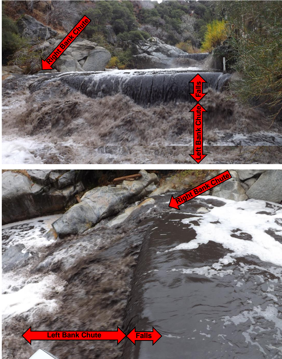
Figure C-6. TOP: Image of project barrier at Kaweah No. 1 Diversion Dam Gage Pool Weir. Kaweah No. 1 Diversion Dam project barrier is visible in background. BOTTOM: Image across width of project barrier at Kaweah No. 1 Diversion Dam Gage Pool Weir towards the right bank.
