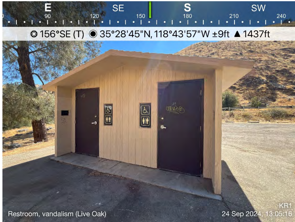
Photo B-70. Live Oak Day Use Area – Pit Toilets
