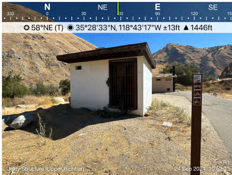
Photo B-29. Upper Richbar Day Use Area – Locked Utility Structure
