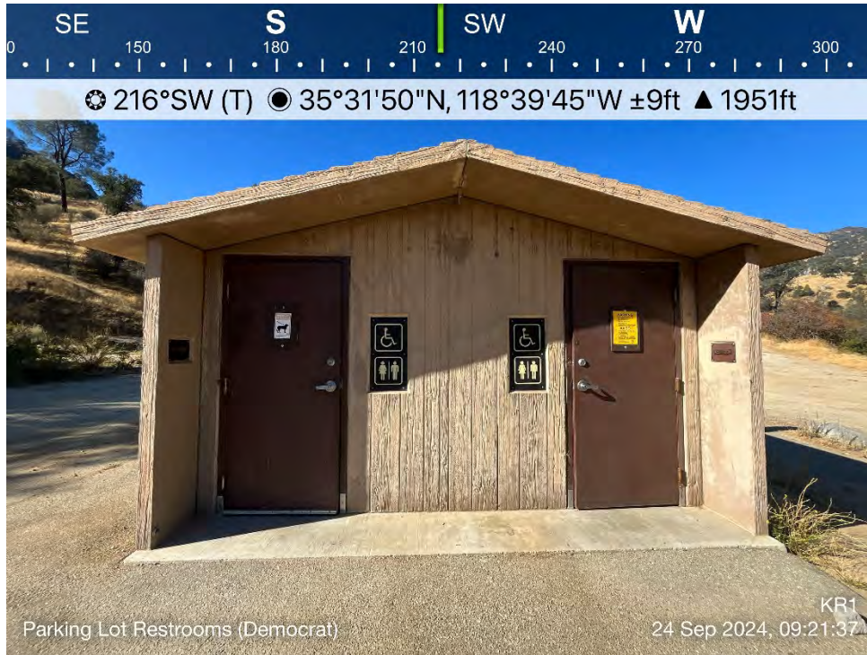
Photo B-7. Democrat Raft Take-out Boating Site – Pit Toilets
