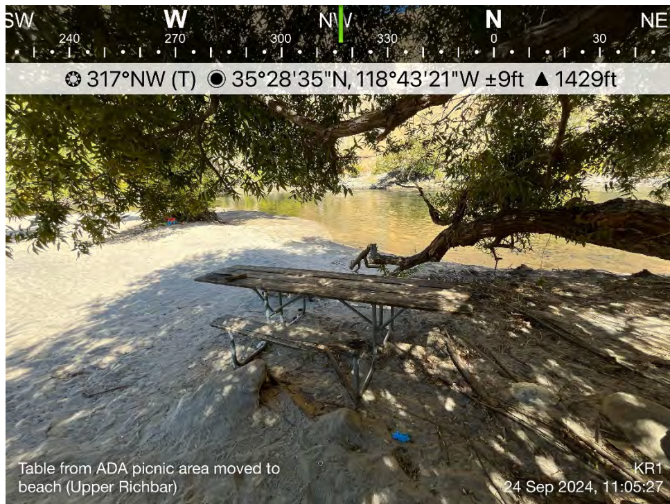
Photo B-39. Upper Richbar Day Use Area – Moved and Damaged FSORAG Compliant Picnic Table
