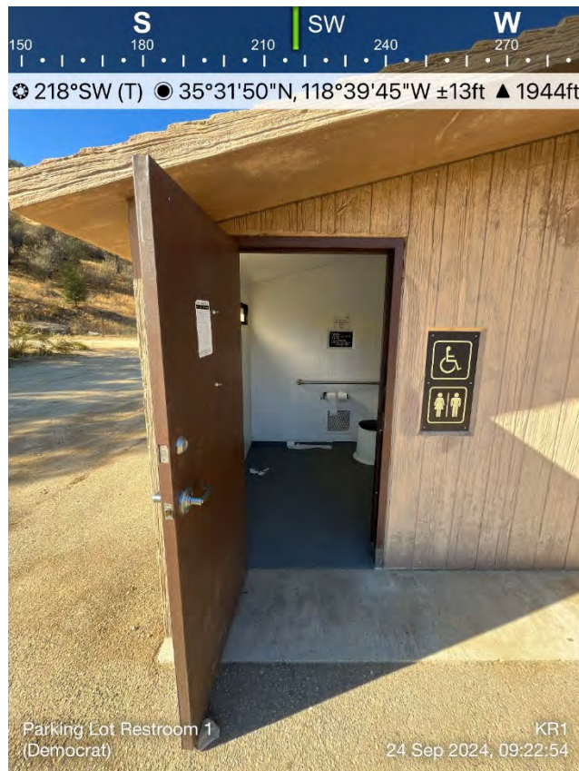
Photo B-8. Democrat Raft Take-out Boating Site – Pit Toilet, Stall 1
