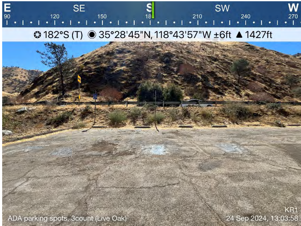
Photo B-68. Live Oak Day Use Area – ADA Parking Spots
