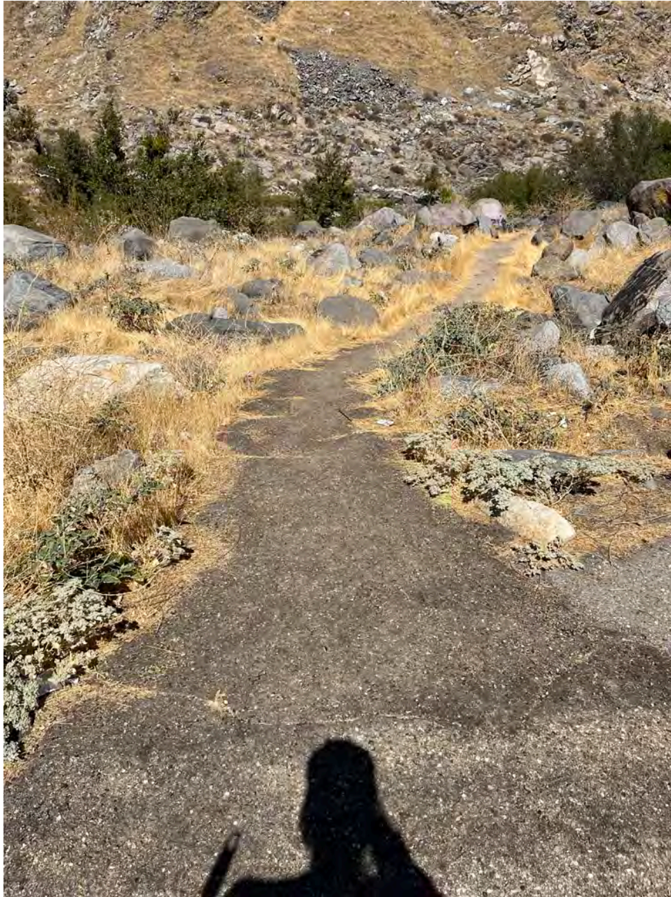
Photo B-77. Live Oak Day Use Area – Paved Access Path
