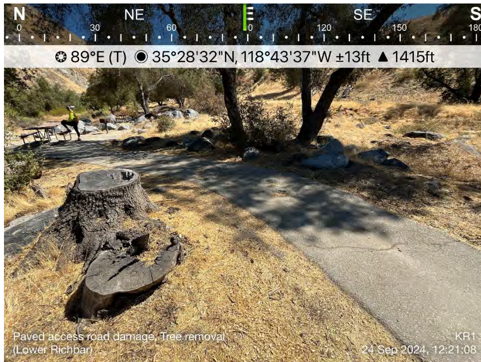
Photo B-60. Lower Richbar Day Use Area – Paved Access Path
