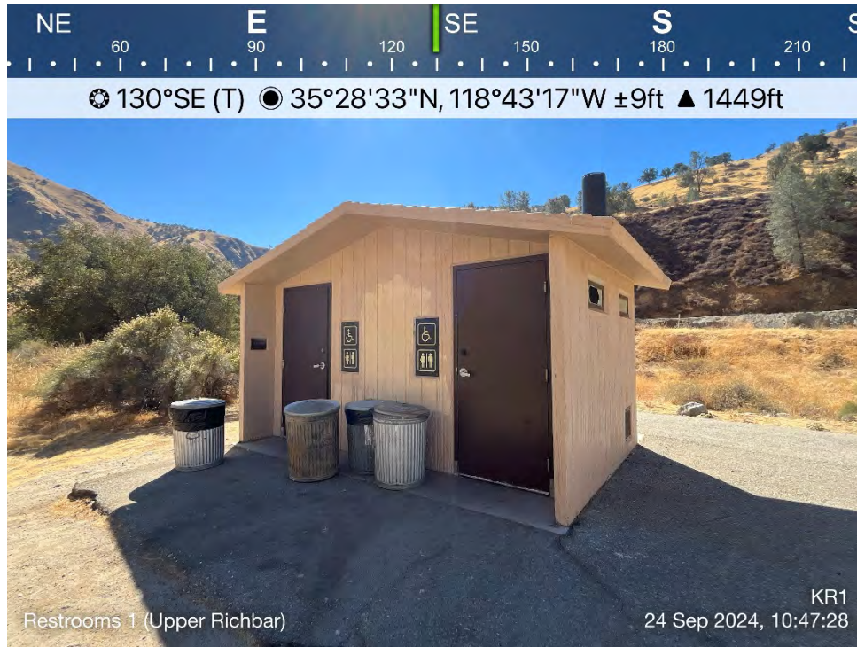
Photo B-30. Upper Richbar Day Use Area – Pit Toilets #1
