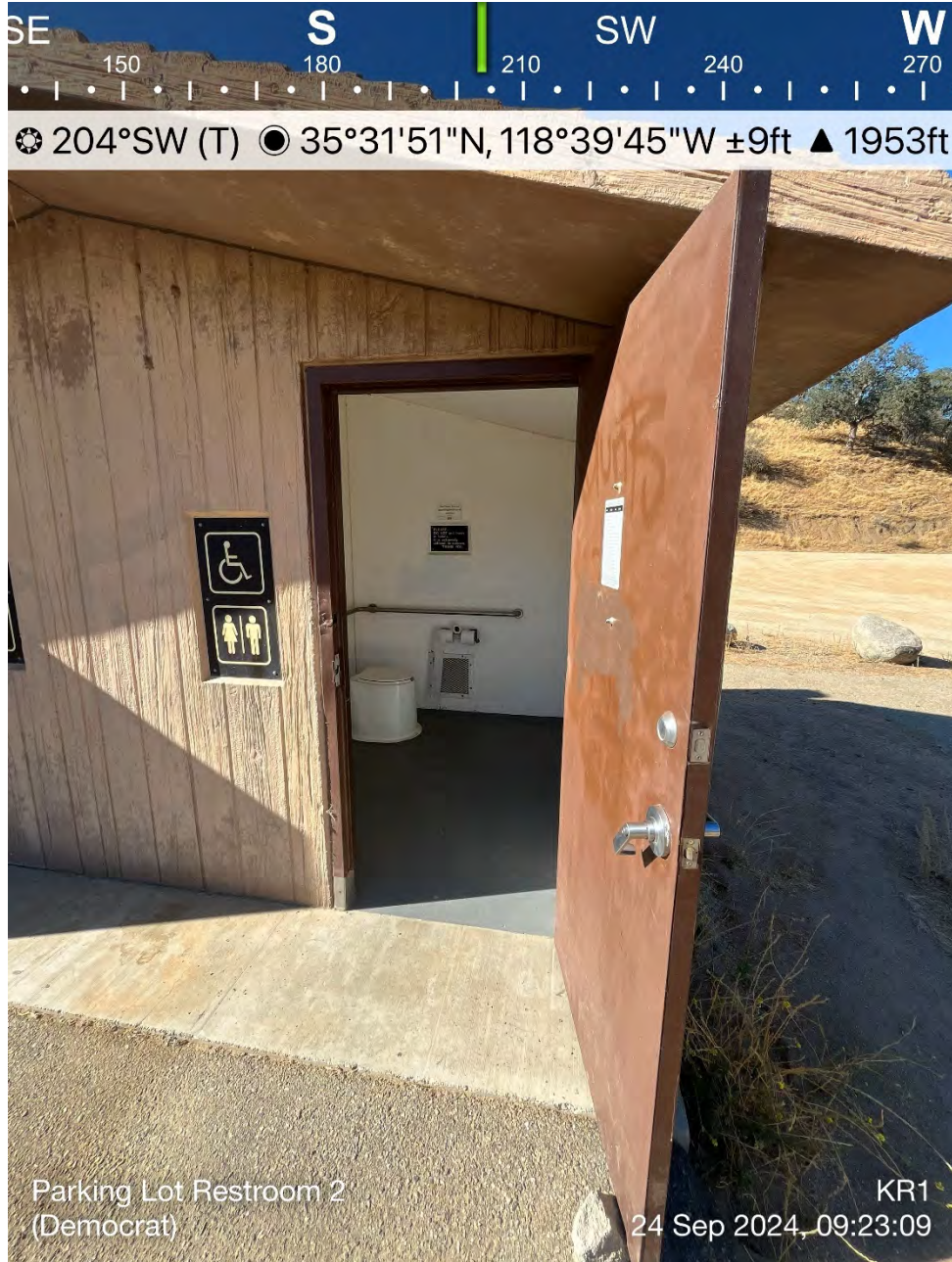
Photo B-9. Democrat Raft Take-out Boating Site – Pit Toilet, Stall 2
