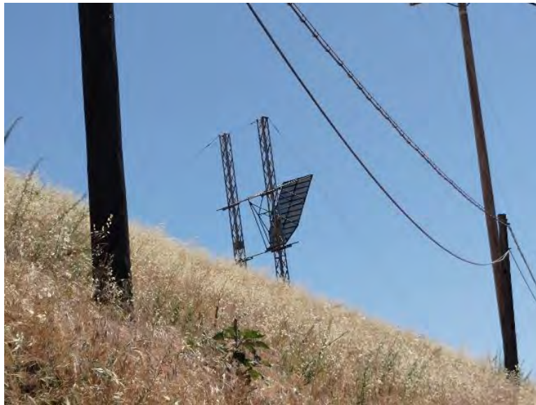
Photo G-26. Communication Site: The metal structure is highly exposed to the elements and lacks suitable roosting areas.
