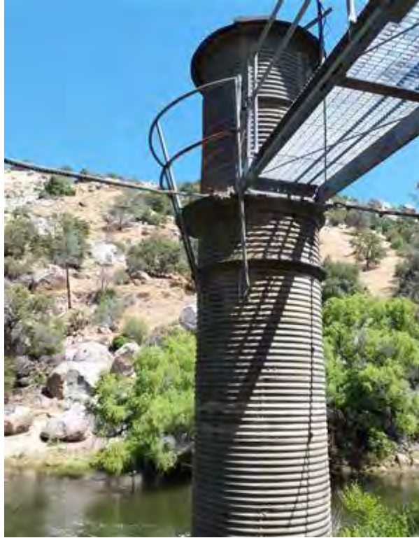
Photo G-9. Stilling Well No. 1: Stilling well has some vertical and roofed elements but is composed of cold, slick steel. This facility is not suitable for roosting.
