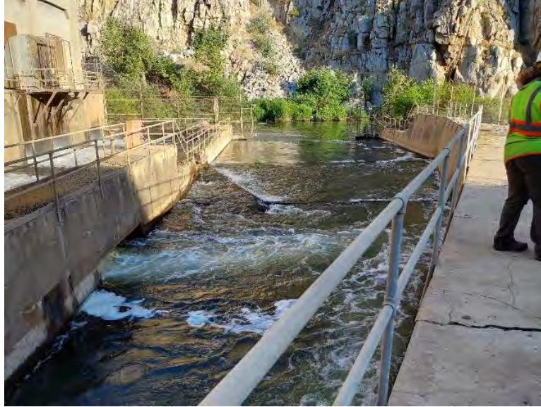
Photo G-29. Trailrace: The tailrace does not support suitable bat roost habitat. It is an open waterway and does not contain roosting elements though bats may drink from it.
