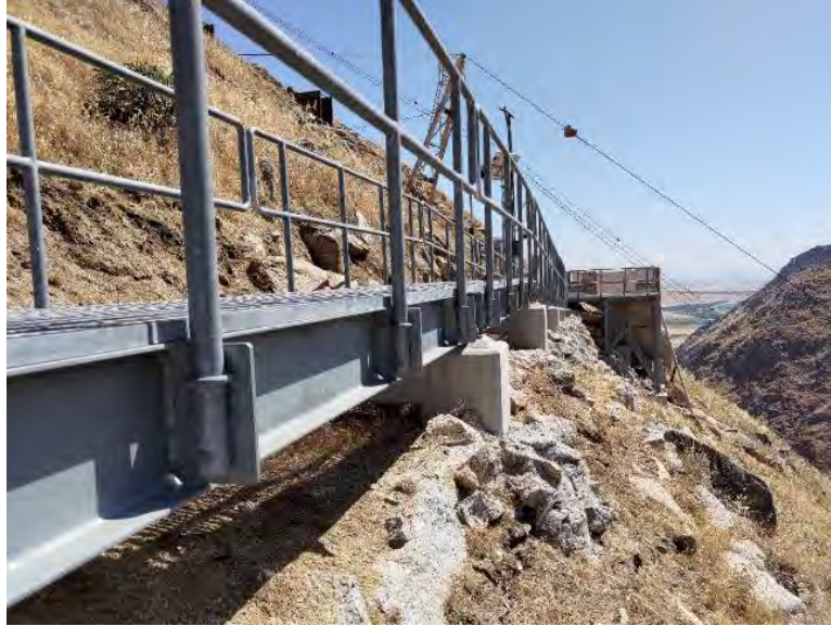
Photo G-27. Skip Hoist Upper Landing and Hoist Cable: The facility has vertical metal structures and a grated walkway. However, it is fully exposed to sun and high winds. The facility is not suitable for roosting.
