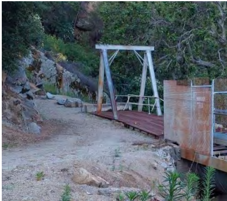
Photo G-8. Conduit No. 2: This conduit has vertical steel segments and roofed a metal crossbeam. However, the metal is not suitable for bats and the high water levels and fast flow within the facility is not suitable for bat roosting.
