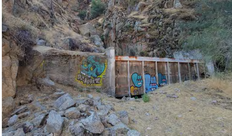
Photo G-13. Conduit No. 4/Conduit No. 5: The conduits are directly up and downstream of the flume have vertical structures but lack roofed elements or entry points for cover during roosting. These facilities are not suitable for roosting.
