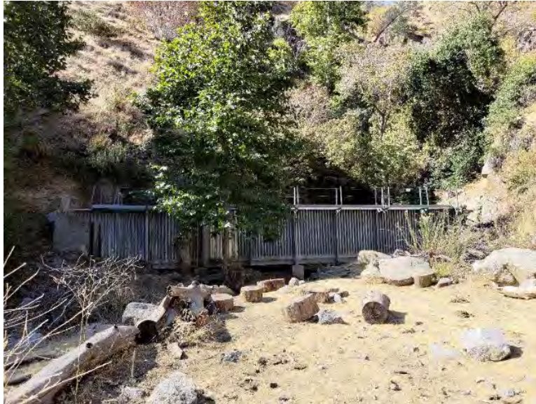
Photo G-17. Flume No. 5 Dougherty Creek/Conduit No. 7: The flume is made of metal and has steel roofed elements that bats could utilize for roosting under appropriate conditions. It also has concrete in some areas which could be used for roosting. The flume could be utilized for roosting if swallow mud nests are present as was observed on Flume No. 4 (Lucas Creek). Bats are not currently utilizing this facility.
