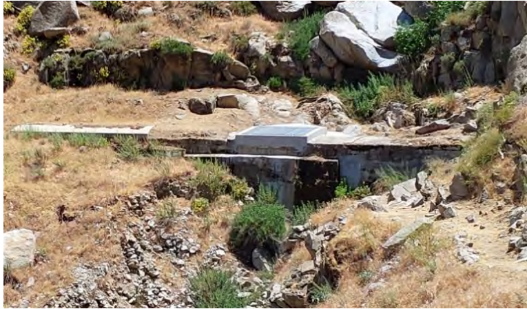
Photo G-23. Conduit No. 9: The concrete structure has a metal covering that bats could enter but it contains flowing water and is not suitable roosting habitat. The exterior has no cracks or crevices. The facility is not suitable for roosting.
