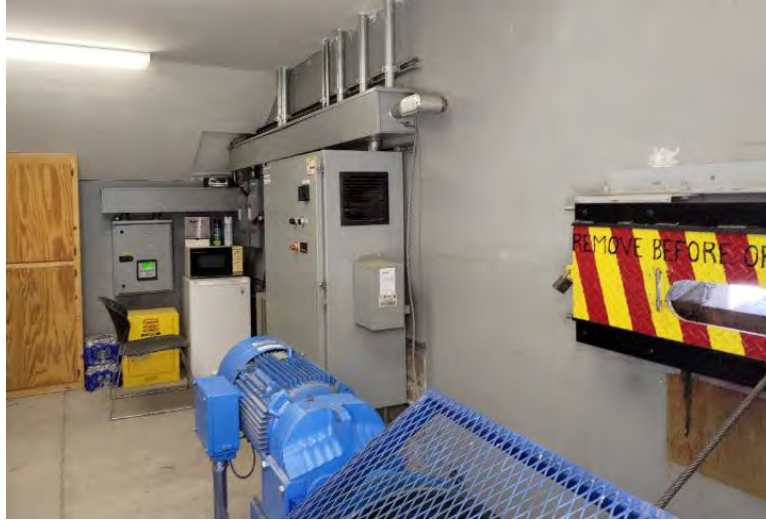
Photo G-33. Skip Hoist House and Lower Landing: The exterior of structure has roofed elements and vertical portions that could be suitable for bat roosts. There are no good entry points for bats. Bats are not currently utilizing this facility.
