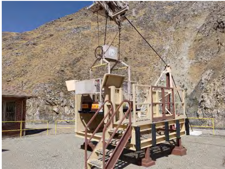
Photo G-32. Aerial Cable Tower and Aerial Cable: The aerial cable tower does not represent appropriate bat roost habitat.
