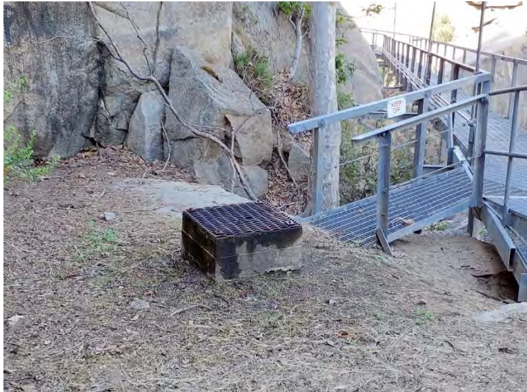
Photo C-2. Conduit No. 1: Not accessible to wildlife. The majority of the facility is underground with one raised grate covered concrete section.
