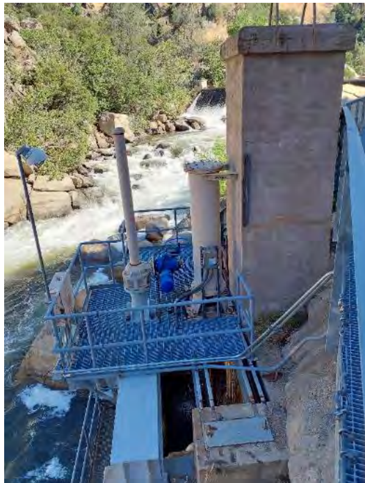
Photo G-4. Drainage Tunnel Outlet: The drainage tunnel outlet is a textured concrete structure with some vertical steel, and roofed elements. This structure could act as a potential night roost. No guano or signs of roosting were observed. This facility is not currently being utilized by bats.
