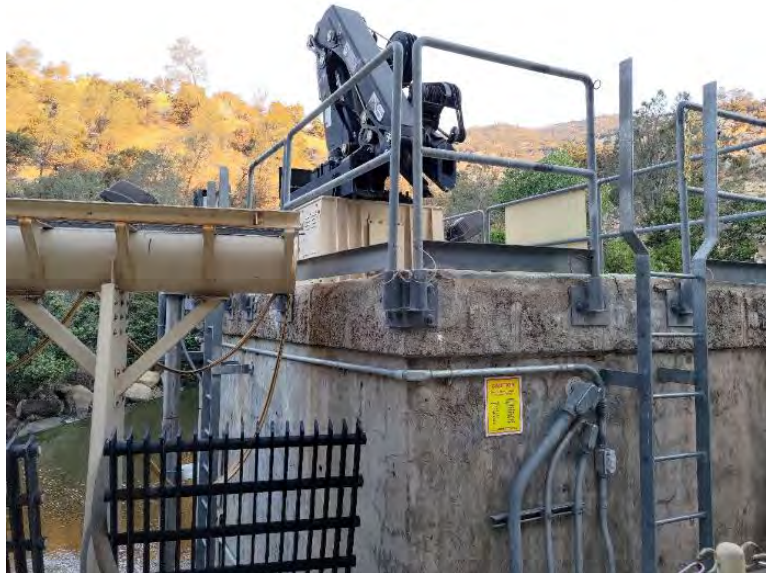
Photo G-2. Drainage Tower: The drainage tower is constructed of vertical steel, some roofed elements, with a concrete material base. However, the structure is too exposed and there are no ways for bats to enter the interior. It is not suitable for roosting.
