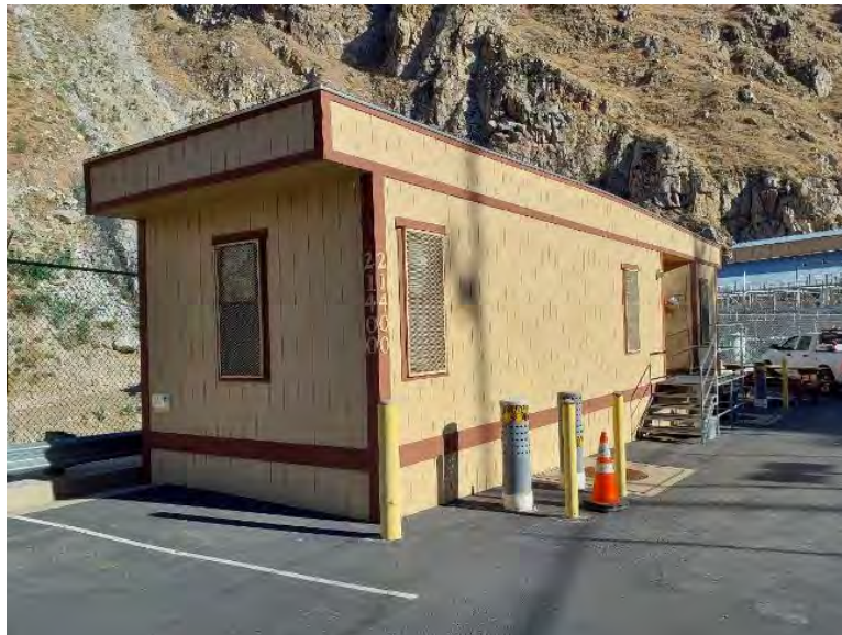
Photo G-40. Office/Lunchroom: The inside of the structure is well-sealed and likely not utilized by bats. The external roofed/vertical portions may have potential for bats to roost overnight. No roost is present. Bats are not currently utilizing this facility.
