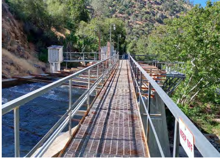
Photo G-5: Democrat Dam Access Walkway: The grated walkway is composed of steel and is exposed. It is not suitable habitat for maternity or day roosting. The roofed elements and vertical structures could potentially support bat roosts at night. The unnamed buildings on the walkway were found to have guano and are suitable night roosting habitat. An active western mastiff bat colony is present adjacent to the walkway on a connected rock crevasse.
