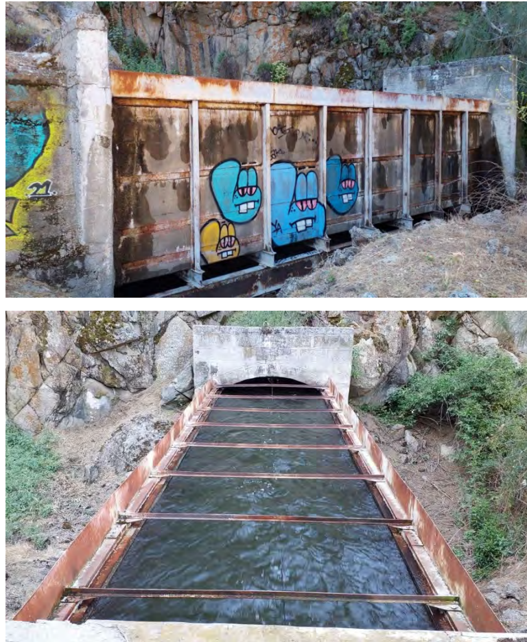
Photo C-7. Flume No. 3: Potentially Accessible to Wildlife. Access to the facility is limited due to the structure's height and metal grate covered walkway. However, open portion of the flume is potentially accessible from the surrounding landscape.
