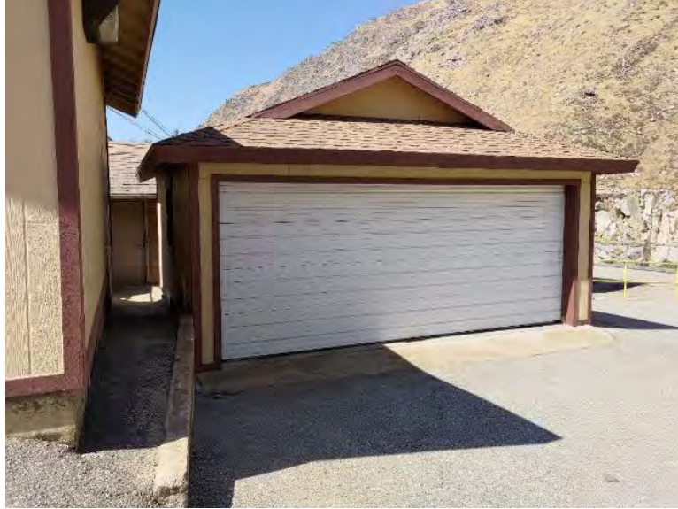
Photo G-35. Garage No. 1: The external portion of this building has roofed elements and some crevices where bats could roost. Not enough guano is present to indicate regular usage but it is likely seasonal night usage while foraging. This facility supports a potential night roost.
