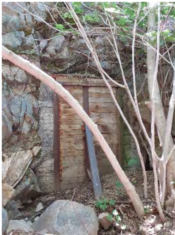
Photo G-20. Adit 12 & 13: The adit has a wooden door/covering and a small roofed element. However, it is too exposed to unfavorable weather conditions and does not contain areas with cover suitable for roosting. The riparian area surrounding adit could be suitable for tree roosting bats.
