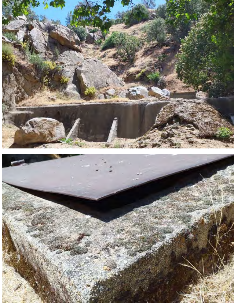
Photo C-5. Conduit No. 3: Not accessible to wildlife. Access to the facility is prevented by existing precautions (i.e., metal covering).
