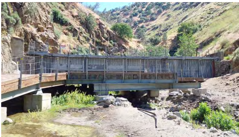
Photo A-7. Stark Creek in the vicinity of Flume No. 6: This location potentially meets the life history requirements for western spadefoot toad. Aquatic breeding habitat was present at the time of the survey and there is suitable upland habitat for adults.
