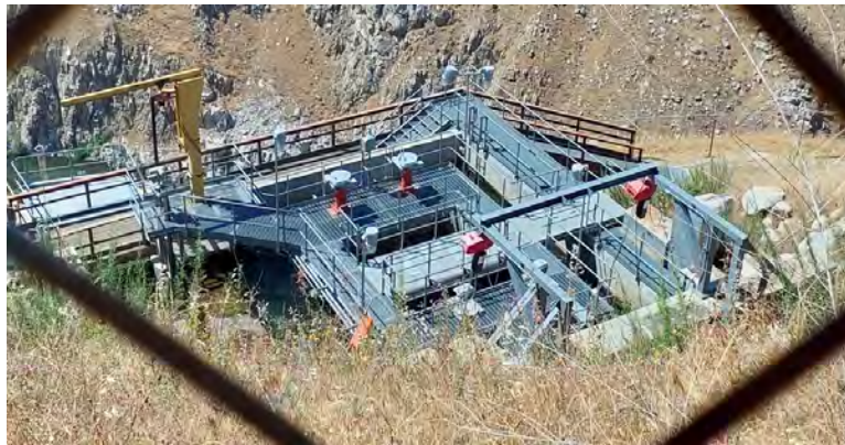
Photo C-13. Forebay: Not accessible to wildlife. Access to the facility is prevented by existing precautions (i.e., perimeter fencing).
