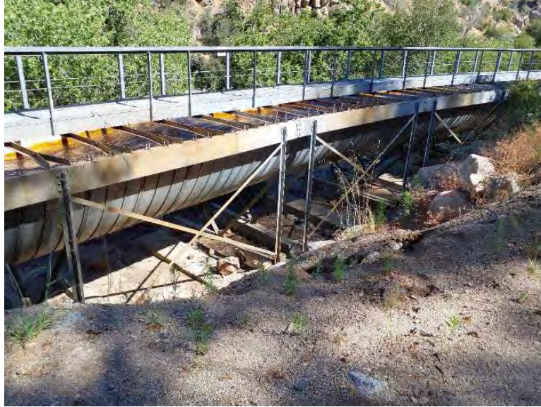
Photo G-7. Flume No. 1: This Project facility supports vertical structures and roofed elements but the vibration from the flow of water and cold metal makes utilization unlikely. This facility is not suitable for roosting.
