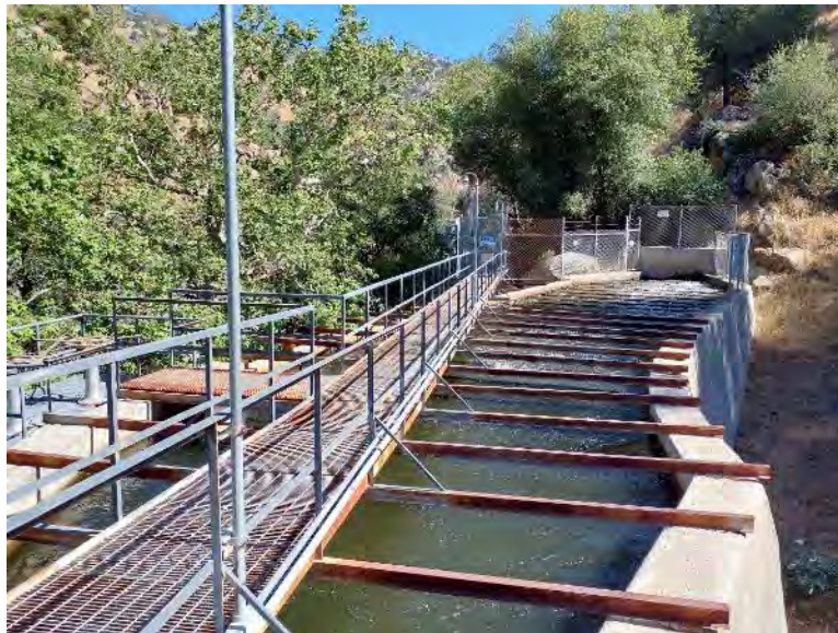
Photo G-6. Sandbox: This Project facility is an open water conveyance system. It is a concrete structure with no cracks or roofed elements that could support bat roosting. This facility is not suitable for roosting.
