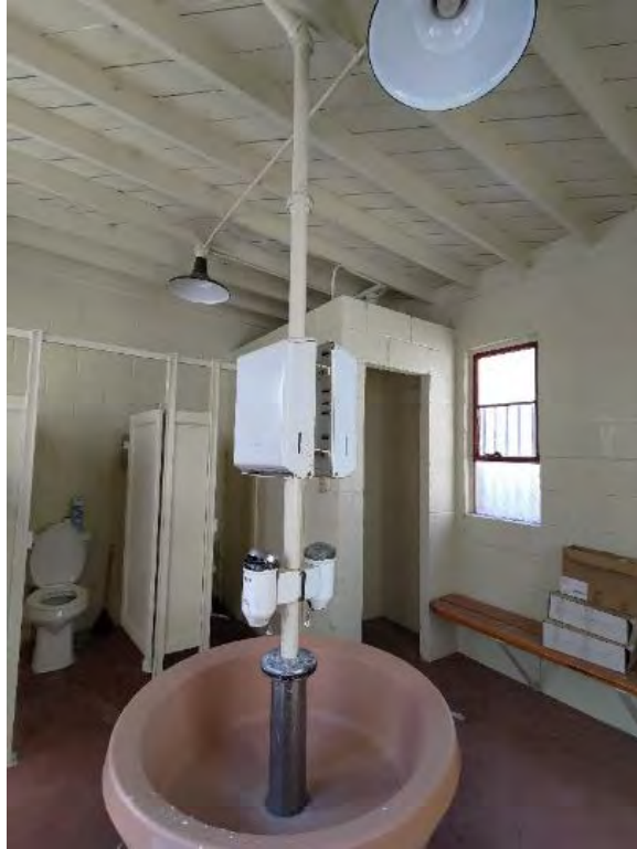
Photo G-39. Restroom: The building contains suitable roosting elements but is well-sealed. No roost is present. Bats are not currently utilizing this facility.
