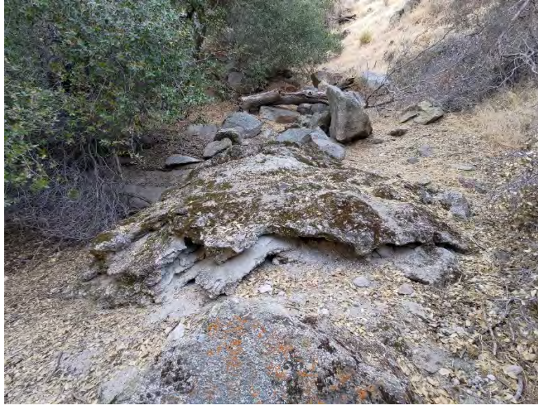
Photo C-8. Conduit No. 6: Not Accessible to Wildlife. The conduit is entirely contained and is not a wildlife risk.
