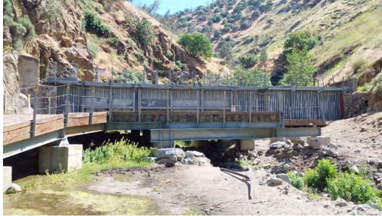
Photo G-19. Flume No. 6 Stark Creek/Conduit No. 8: The flume is made of metal and largely not suitable habitat for roosting bats. The conduit is made of concrete with no cracks or areas that bats could utilize. The flume could be utilized for roosting if swallow mud nests are present as was observed on Flume No. 4 (Lucas Creek).
