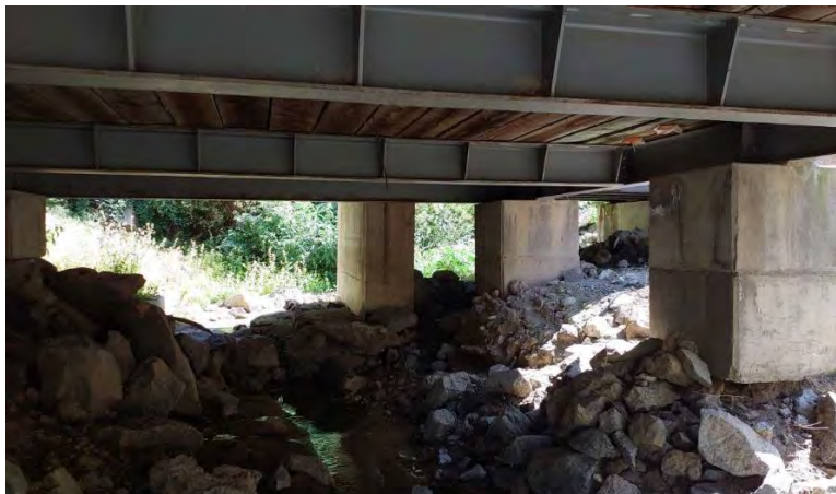
Photo G-18. Access Platform: The underside of the platform is very open with no good roosting locations on metal girders and wooden planks where bats could be sheltered. Cattle also often disturb this area passing under this location. This facility is not suitable for roosting.
