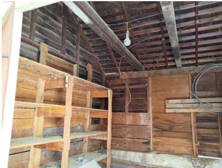
Photo G-34. Old Icehouse: The exterior of structure has roofed elements and vertical portions that could be suitable for bat roosts. There are no good entry points for bats. Bats are not currently utilizing this facility.
