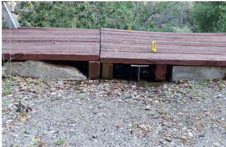
Photo C-4. Conduit No. 2: Not accessible to wildlife. The small segment of conduit adjacent to Flume No. 1 is covered/fenced to prevent access.
