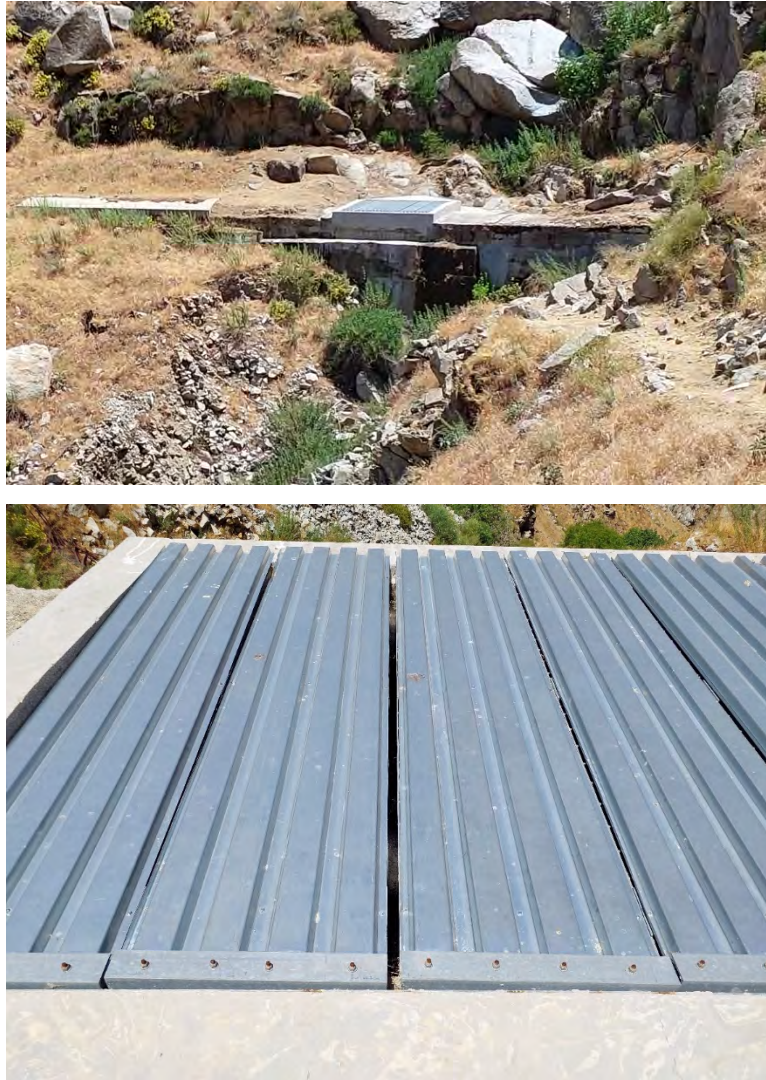
Photo C-12. Conduit No. 9: Not accessible to wildlife. Access to the facility is prevented by existing precautions (i.e., metal covering).
