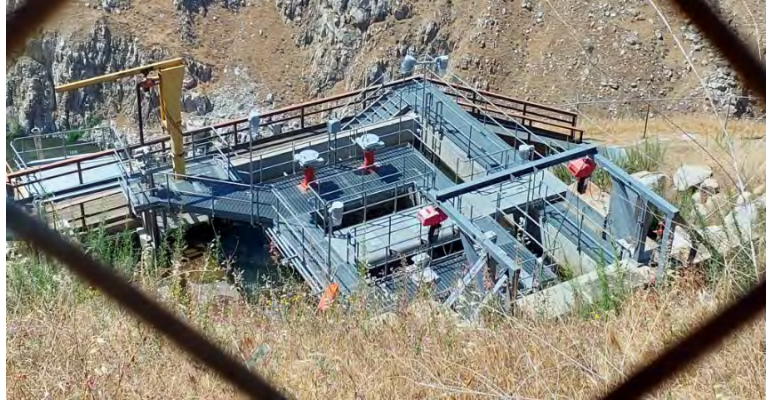
Photo G-25. Forebay: The forebay is an open water conveyance system with steel grates and structures over the top. The structure is fully exposed to the sun and there are high winds. The facility is not suitable roosting habitat but could be used for foraging or hydration.
