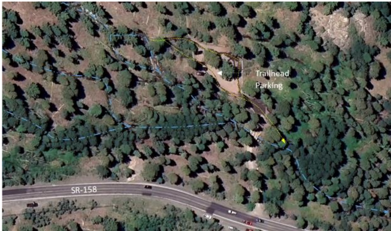
Photo AQ 5-40. Example location where overbank flows from Fern Creek (blue lines) are eroding the Fern/Yost trailhead parking area and re-entering the creek downstream of the bridge (yellow lines).
