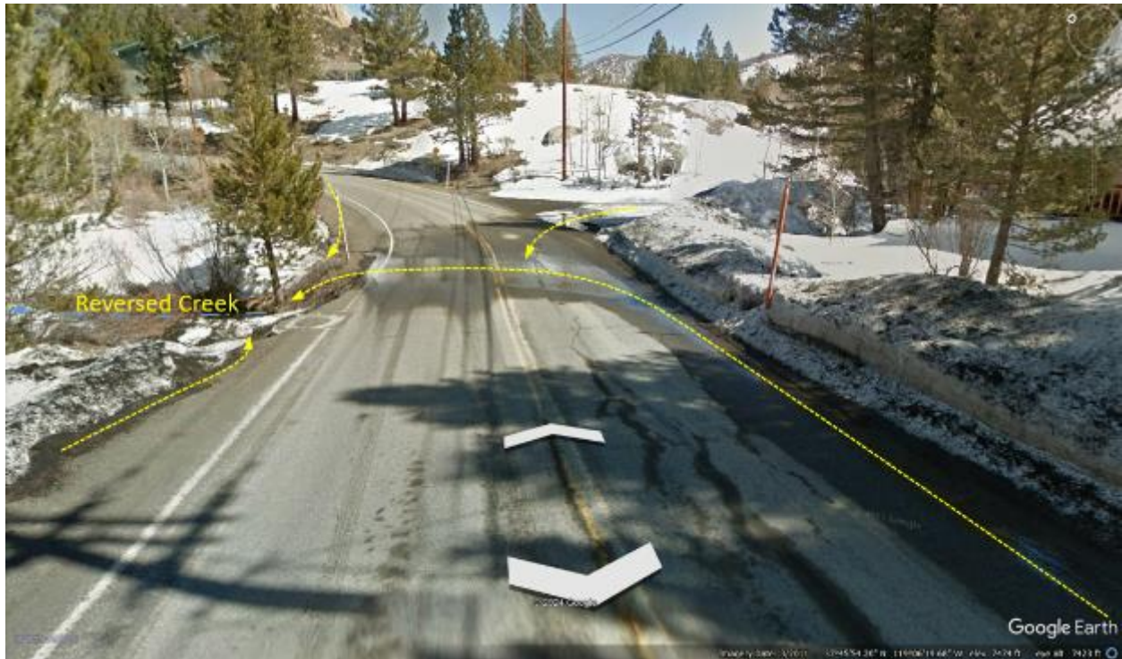
Photo AQ 5-41. Google street view photo showing an example of road runoff from SR-158 (and spur roads) entering directly into Reversed Creek carrying with it sediment from sanding the roadway.
