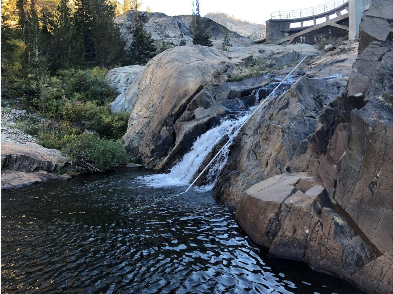
FP5A (Cascade below Agnew Dam Outlets) – An approximately 13-foot-high cascade barrier, shown with 25-foot rod for size reference, occurs immediately below Agnew Dam. This cascade prevents fish from reaching the base of Agnew Dam. Brook trout were observed in the field attempting, and failing, to ascend this barrier.
