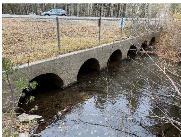
Highway 158 Crossing – Analysis indicates this culvert crossing does not present a barrier to fish movement.
