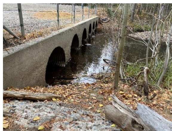
Highway 158 Crossing – Analysis indicates this culvert crossing does not present a barrier to fish movement.
