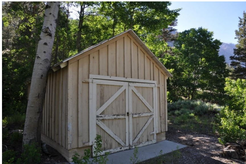
Photo 43. Rush Creek Powerhouse Building 0113. This facility was determined to be suitable bat roosting habitat. Building provides vertical and roofed components that could potentially support roosting bats. The building has cracks and crevices that bats could enter, and the building has appropriate thermal conditions (high solar exposure).
