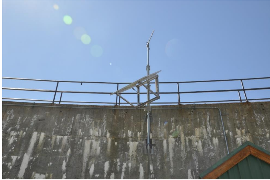
Photo 15. Rush Meadows Dam Solar Facility. This facility is unsuitable for bat roosting. Metal structure does not contain suitable overhangs or crevices for bat roosting.
