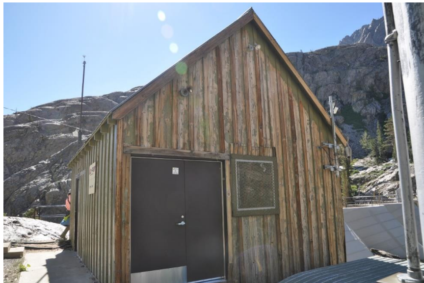
Photo 31. Lower Agnew Lake Boathouse/Dock. This facility was determined to be suitable bat roosting habitat. The building contains holes for bats to enter and suitable solar exposure. The cracks in the corrugated metal roof could also provide suitable entrance points for roosting.
