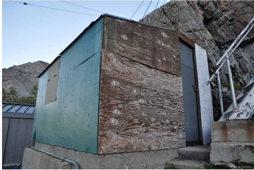
Photo 23. Gem Dam Overhead Hoist House for Dam Length. This facility was determined to be suitable bat roosting habitat. Wooden building with holes that bat could potentially access suitable roosting habitat.
