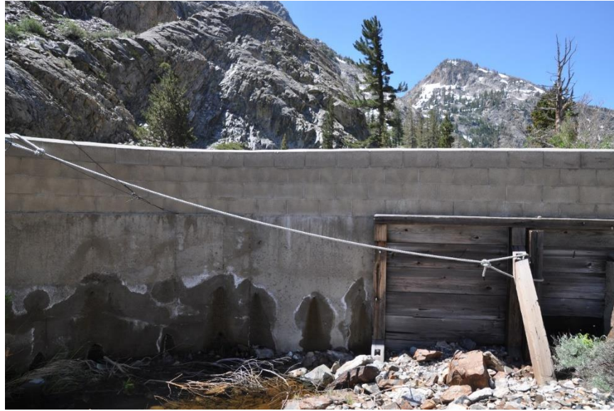
Photo 35. Agnew Flume (downstream of Agnew Dam). This facility is unsuitable for bat roosting. The flume is made of relatively new concrete that does not have cracks and crevices for bats to enter and lacks roofed elements. The flume conveys Rush Creek which makes the walls of the structure too cold for day roosting.
