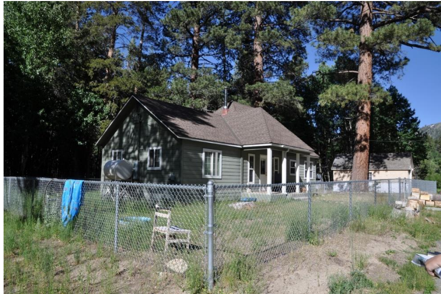
Photo 36. Rush Creek Powerhouse Cottage No. 1. This facility was determined to be suitable bat roosting habitat. Bats could potentially roost under roof eaves on the building. There may be a few cracks under the shingles for bats to access the interior. Building receives solar exposure.
