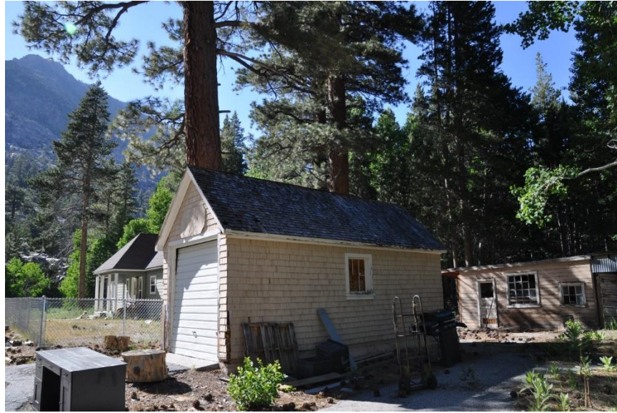
Photo 37. Rush Creek Powerhouse Garage No. 1. This facility was determined to be suitable bat roosting habitat. Structure contains vertical and roofed components and cracks and crevices suitable for bat roosting. Building has appropriate thermal conditions (high solar exposure).
