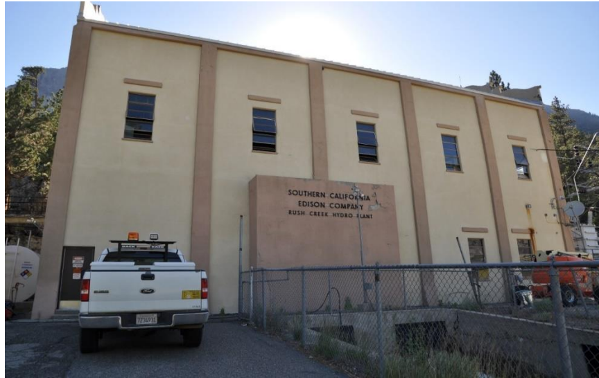
Photo 60. Rush Creek Powerhouse. This facility was determined to be suitable bat roosting habitat. Building provides vertical and roofed components that could potentially support roosting bats. The building has cracks and crevices where bats could enter the facility. The building has appropriate thermal conditions for maternity roosting (high solar exposure).
