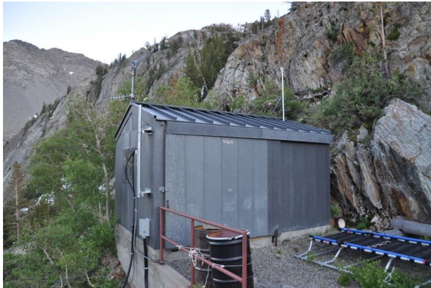
Photo 22. Gem Dam Storage Shed. This facility was determined to be suitable bat roosting habitat. Metal building does not provide suitable bat roosting habitat, but the pipe opening provides a large enough crevice for some smaller bat species to roost. The building has appropriate thermal conditions for maternity roosting (high solar exposure).
