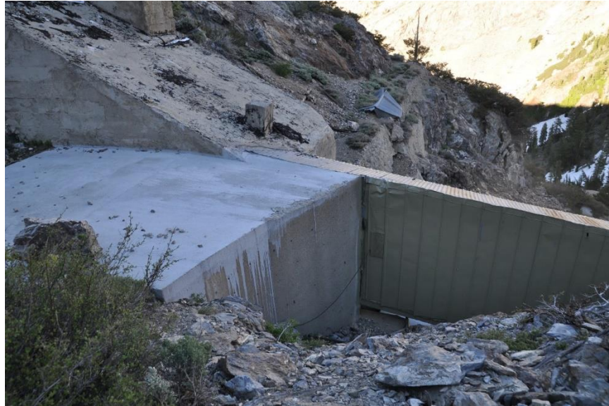
Photo 30. Gem Valve House Tunnel. This facility is unsuitable for bat roosting. The tunnel is used as a spillway during high flows. The concrete pad does not contain roofed elements or cracks and crevices suitable for roosting and the conveyance of water makes this structure unsuitable.
