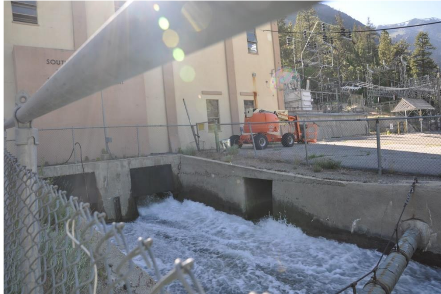
Photo 49. Rush Creek Powerhouse Tailrace. This facility is unsuitable for bat roosting. A tailrace is a cold, fast, flowing channel of water out of the powerhouse which would not provide suitable bat roosting habitat.
