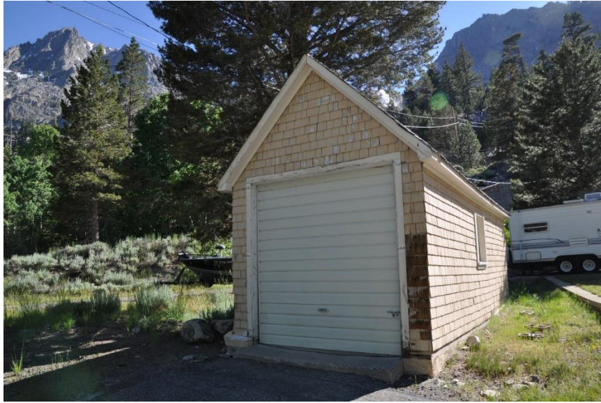
Photo 39. Rush Creek Powerhouse Garage No. 2. This facility was determined to be suitable bat roosting habitat. Building provides vertical and roofed components that could potentially support roosting bats. The building has cracks and crevices that bats could enter and the building has appropriate thermal conditions (high solar exposure).
