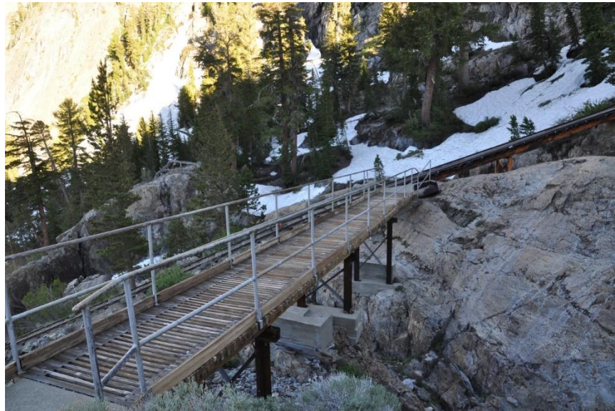
Photo 26. Gem Tram Landing Footbridge. This facility was determined to be suitable bat roosting habitat. Open slatted wood provides roofed elements for roosting, but structure lacks tight cracks and crevices and is very open to the air. Location receives suitable solar exposure for day roosting.
