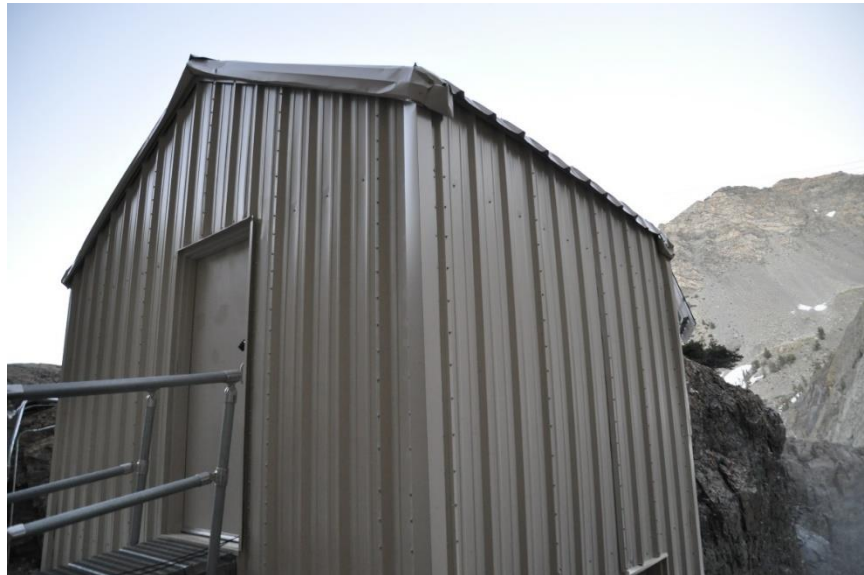
Photo 6. Gem Dam Arch 8 Valve House. This facility is unsuitable for bat roosting. This metal building has no cracks, crevices, or entry points for bats. Roofed elements are made of metal, which do not provide a suitable gripping surface for roosting.
