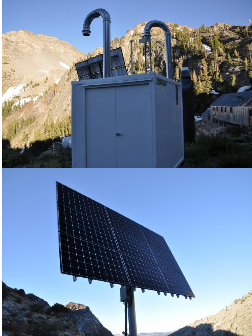
Photo 29. Gem Satellite Dish/ Gem Solar Facility. This facility is unsuitable for bat roosting. The satellite dish and solar facility do not provide roofed elements or cracks and crevices suitable roosting habitat. The building that is connected to the satellite dish/solar facility has no openings for bats to enter.
