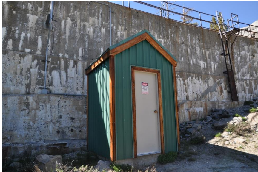
Photo 14. Rush Meadows Dam Gage House. This facility was determined to be suitable bat roosting habitat. Building contains wooden overhangs under which bats could roost, but lacks cracks and crevices allowing access to the interior.
