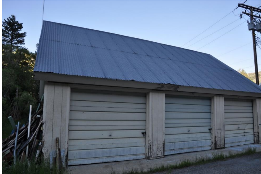
Photo 41. Rush Creek Powerhouse Garage No. 4. This facility was determined to be suitable bat roosting habitat. Building provides vertical and roofed components that could potentially support roosting bats. The building has cracks and crevices where bats could enter the building has appropriate thermal conditions (high solar exposure).
