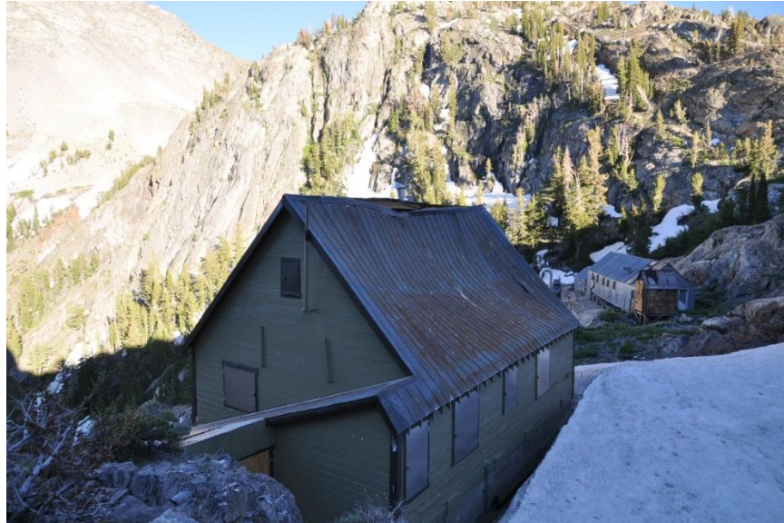
Photo 5. Gem Valve House and Cabin. This facility was determined to be suitable bat roosting habitat. This wooden building has openings along the tin roof and cracks around windows where bats could enter. Building receives appropriate solar exposure.
