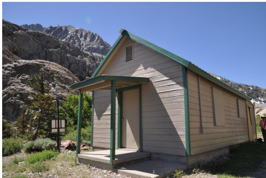
Photo 34. Agnew Cabin. This facility was determined to be suitable bat roosting habitat. Building provides vertical and roofed components that could potentially support roosting bats. The building has cracks and crevices where bats could enter. Building is located in an area that has appropriate thermal conditions for maternity roosting (high solar exposure).
