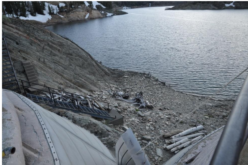
Photo 16. Gem Lake Dock. This facility is unsuitable for bat roosting. This is a concrete slab close to the ground and water. There is no overhangs or cracks and crevices for roosting.
