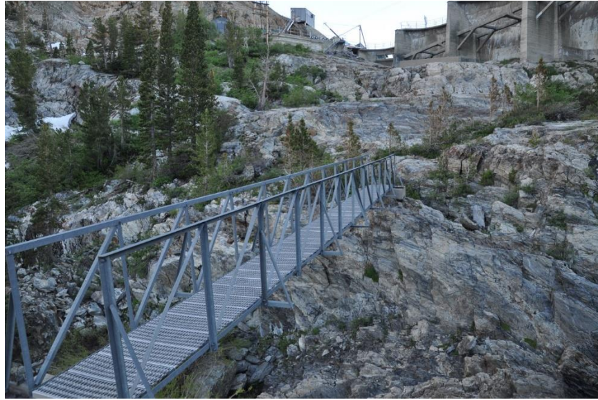
Photo 25. Gem Fish Release Footbridge. This facility is unsuitable for bat roosting. Metal grating bridge that stretches over Rush Creek does not provide roofed elements or cracks and crevices suitable for roosting. Metal material does not provide a suitable gripping surface.
