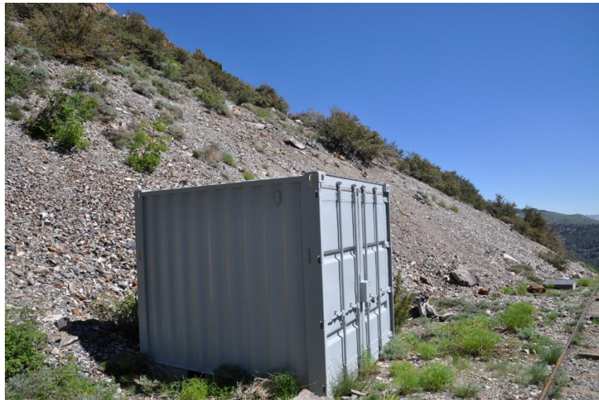
Photo 59. Agnew Tram Landing (metal storage building not identified on facility list or on the maps). This facility is unsuitable for bat roosting. Metal storage container does not provide roofed components or cracks and crevices that could potentially support roosting bats.
