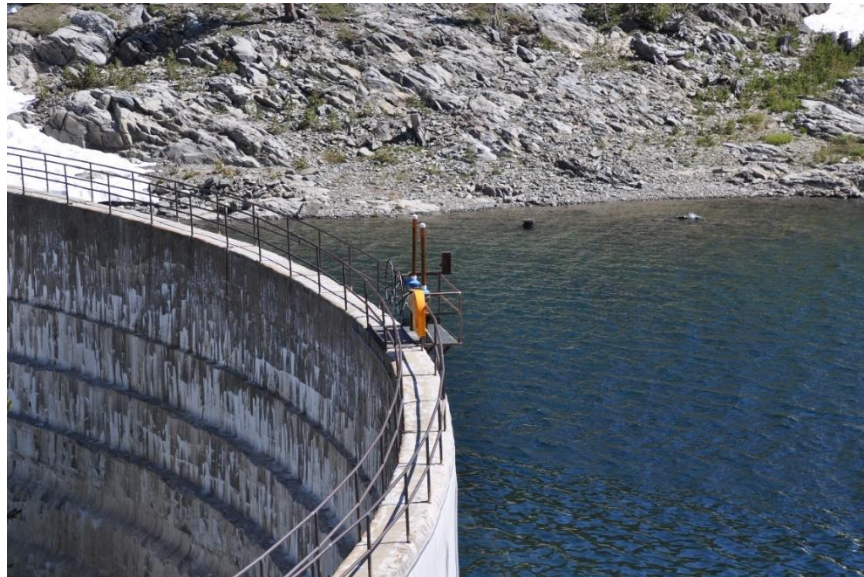
Photo 4. Rush Meadows Dam Valve House. This facility is unsuitable for bat roosting. The valve house does not have overhangs or crevices suitable for bat roosting. Valve house is partially inundated with water and does not have appropriate thermal conditions.
