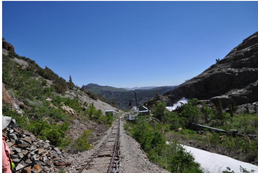
Photo 57. Agnew Tram. This facility is unsuitable for bat roosting. Tram line does not provide vertical or roofed components that provide appropriate bat roosting habitat. Tram line lies against the ground.
