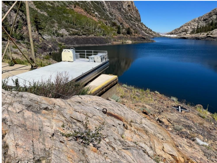
Photo 32b. Upper Agnew Lake Dock. This facility was determined to be suitable bat roosting habitat. The dock contains suitable wooden roofed elements with corrugated metal sheeting that provides cracks and crevices for bats to access the interior. The concrete pad where the building sits also has a wooden edge that also provide roofed elements.
