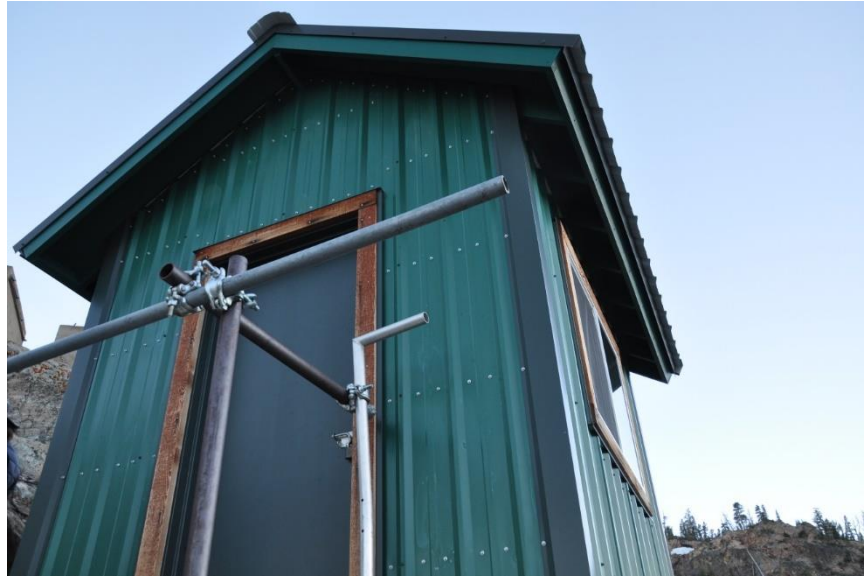
Photo 21. Gem Dam Compressor Shed. This facility is unsuitable for bat roosting. New metal building with no gaps in door or along roofline. There are metal eaves do not provide a suitable gripping surface for bat roosting (i.e., lacks cracks and crevices for bats to grip).
