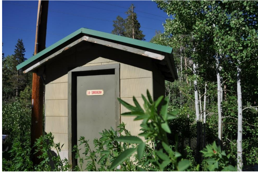
Photo 51. Unnamed Shed near Rush Creek Powerhouse. This facility was determined to be suitable bat roosting habitat. Building provides vertical and roofed components that could potentially support roosting bats. Cracks and crevices on the shingle siding may provide openings for small bats. Building has appropriate thermal conditions for maternity roosting (high solar exposure).
