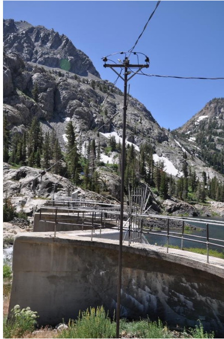
Agnew Lake Dam Powerline. This photograph shows an equipment pole with an insulated guy wire and jumper wires. This configuration does not represent a risk for avian electrocution.
