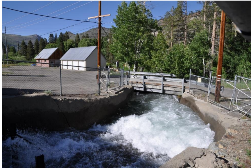
Photo 48. Bridge over Rush Creek Powerhouse Tailrace. This facility is unsuitable for bat roosting. Tailrace water levels are routinely high (to bottom of bridge), which would prevent bat roosting.
