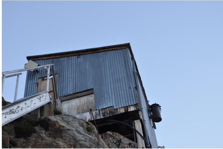
Photo 54. Gem Tram Hoist House. This facility was determined to be suitable bat roosting habitat. Building provides vertical and roofed components that could potentially support roosting bats. The building has cracks and crevices that bats could enter and has appropriate thermal conditions for maternity roosting (high solar exposure).
