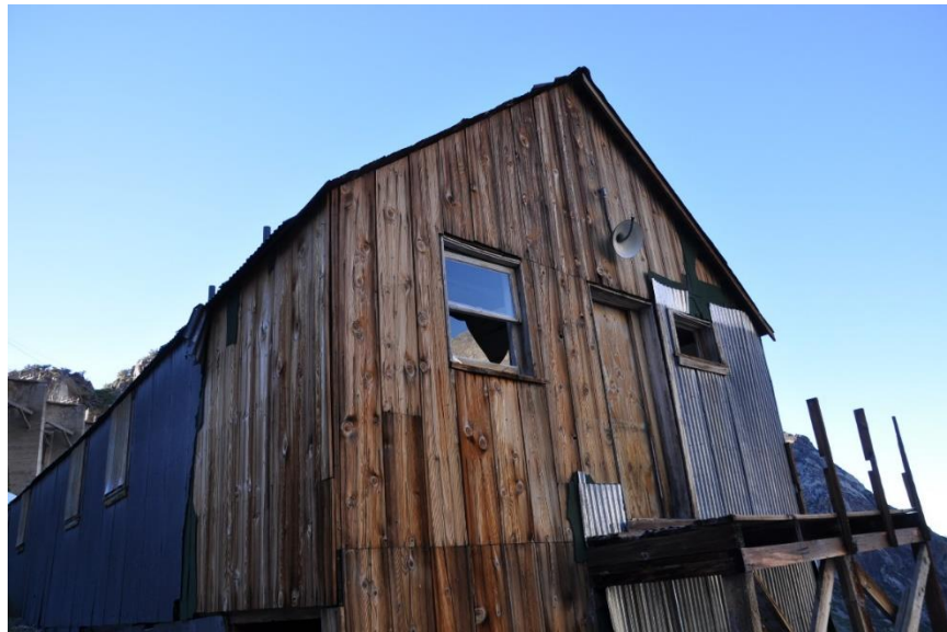
Photo 18. Gem Bunkhouse. This facility was determined to be suitable bat roosting habitat. This building provides suitable roofed elements, cracks, crevices, and open window entrance points for bats. Building is positioned in an area with high solar exposure for maternity roosting.
