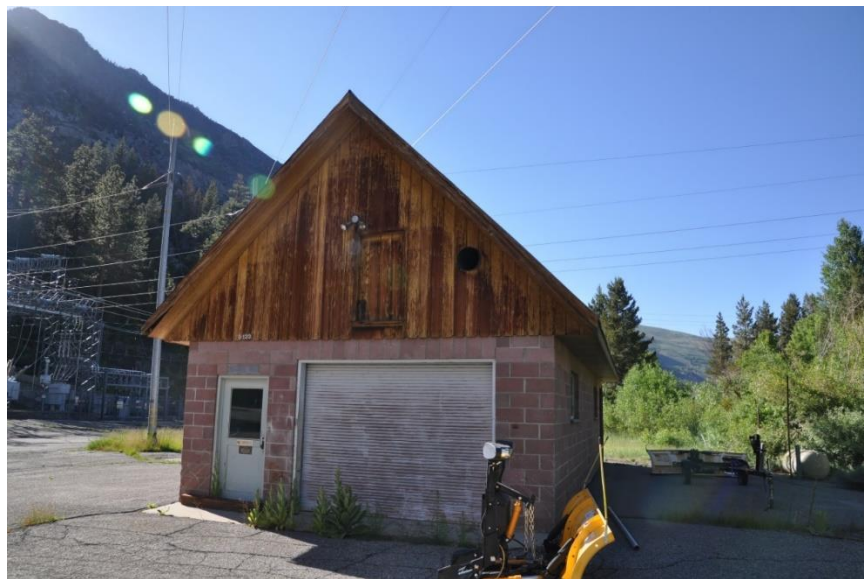
Photo 44. Rush Creek Powerhouse Machine Shop. This facility was determined to be suitable bat roosting habitat. Building provides vertical and roofed components that could potentially support roosting bats. The building has cracks and crevices that bats could enter. The building also provides warm thermal conditions for potential roosting bats.
