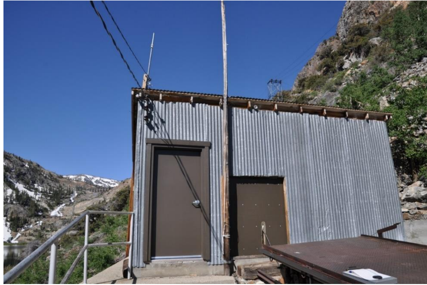
Photo 58. Agnew Tram Hoist House. This facility was determined to be suitable bat roosting habitat. Building provides vertical and roofed components and has cracks and crevices that could potentially support roosting bats. Building has appropriate thermal conditions for maternity roosting (high solar exposure).
