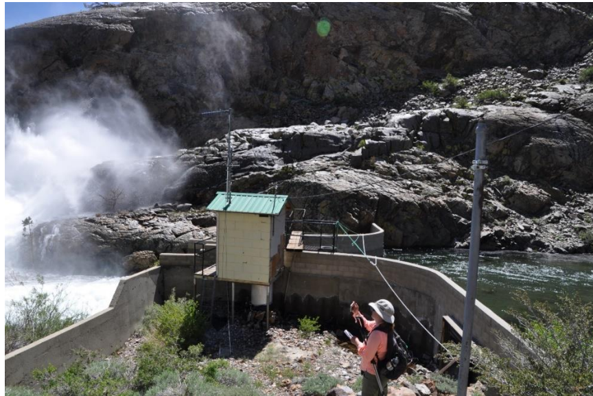
Photo 10. Rush Creek below Agnew Lake (USGS No. 10287289; SCE No. 357). This facility was determined to be suitable bat roosting habitat. The gage building contains suitable cracks and crevices. Underneath the gage is a roofed overhang. Building receives appropriate solar exposure.
