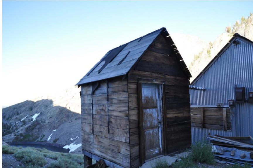
Photo 19. Gem Outhouse. This facility was determined to be suitable bat roosting habitat. This wooden building contains suitable roofed elements, cracks and crevices for bat entry, and is in an area that has appropriate thermal conditions for maternity roosting (high solar exposure).
