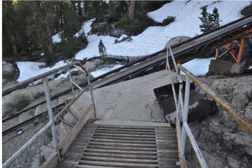
Photo 56. Gem Tram Lower Landing. This facility is unsuitable for bat roosting. Lower landing is a concrete slab on the ground that does not provide vertical or roofed components or cracks/crevices for roosting bats.
