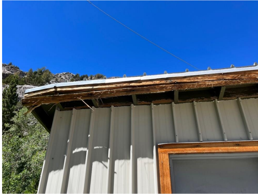
Photo 32a. Upper Agnew Lake Boathouse. This facility was determined to be suitable bat roosting habitat. The building contains suitable wooden roofed elements with corrugated metal sheeting that provides cracks and crevices for bats to access the interior. The concrete pad where the building sits also has a wooden edge that also provide roofed elements. The building has appropriate thermal conditions for maternity roosting (high solar exposure).
