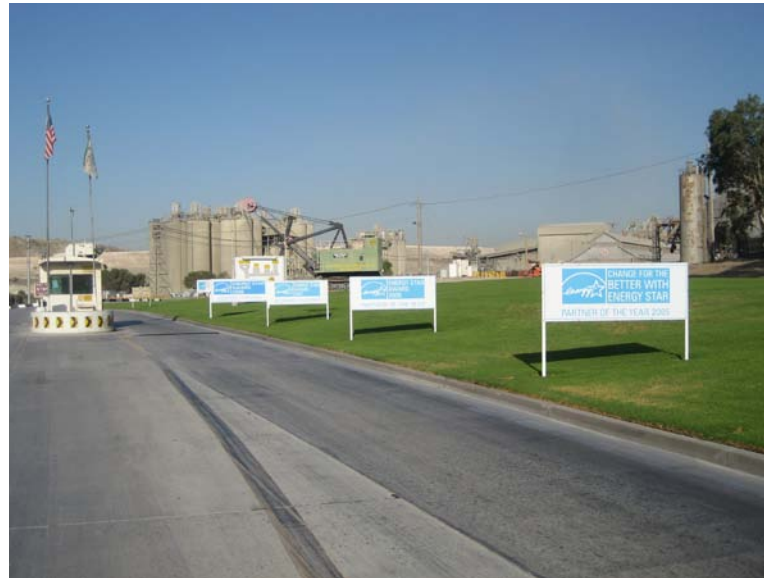
CalPortland Cement Company worked with SCE to identify process improvements leading to potential savings of up to 23.2 million kilowatt-hours at the Colton Cement Plant (shown here) and other local facilities.
