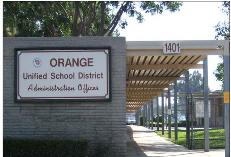
From 2007 through 2009, the Orange Unified School District saved about 3.4 million kilowatt-hours by participating in SCE energy efficiency programs and receiving incentives to upgrade to or install new high-efficiency equipment.
