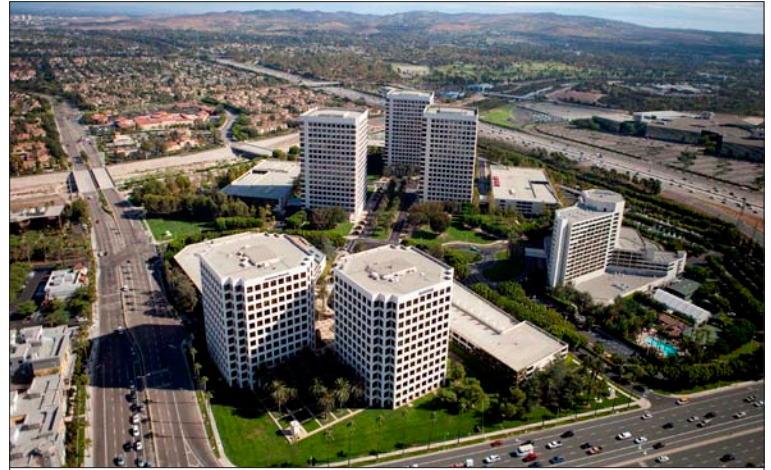
Commercial real estate leader the Irvine Company currently saves 8 million kilowatt-hours annually—approximately $1.2 million—by participating in SCE's energy efficiency programs.
