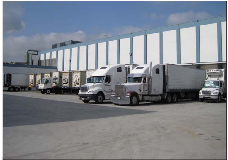
By working with SCE on energy efficiency measures and demand response program participation, Buena Park Cold Storage said it currently saves approximately $200,000 annually on its electricity bill at its frozen foods warehouse.
