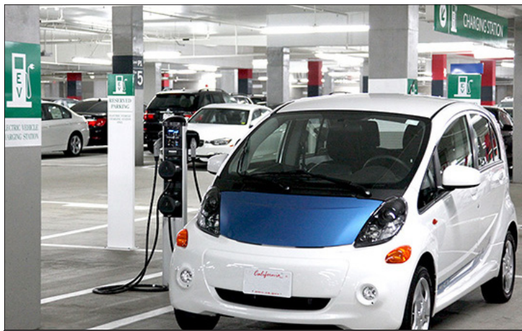
The EV charging stations are located in the center of the parking garage.
