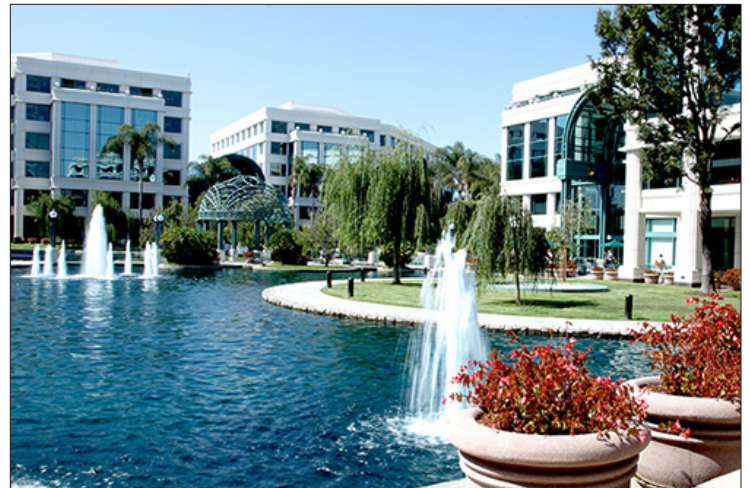
The Water Garden – a 17-acre, Class A office complex in Santa Monica – currently features eight EV charging stations.
