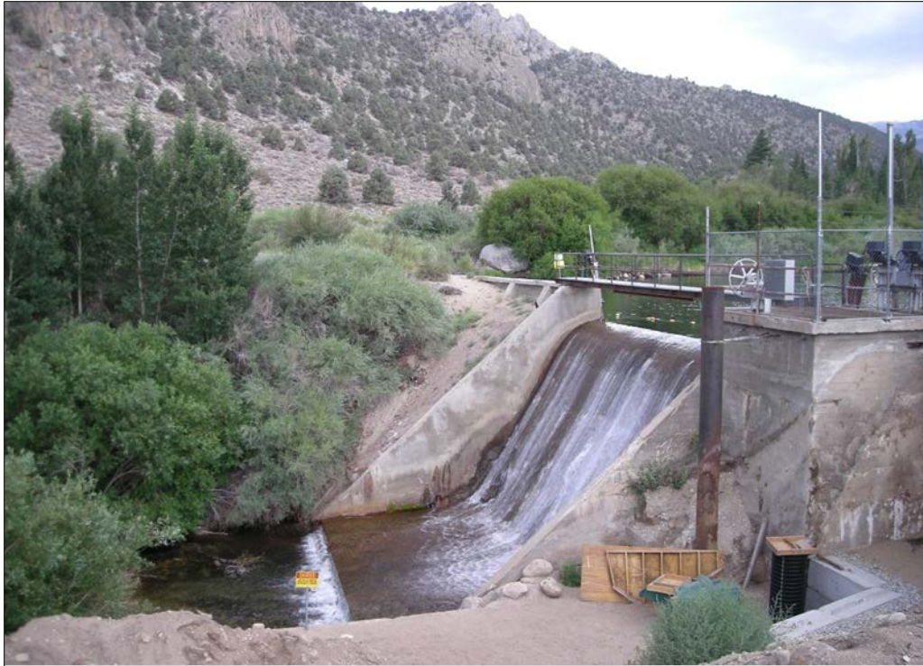
Photo 9.10-9. Plant No. 3 Spillway
