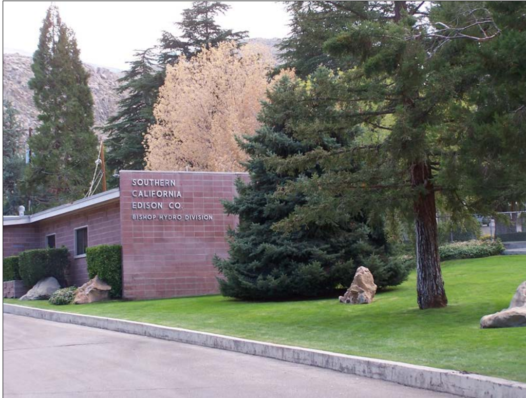
Photo 9.10-7. SCE Office at Plant No. 4
