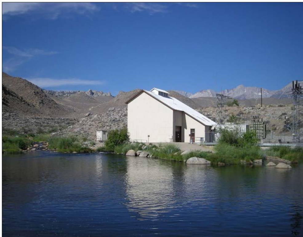
Photo 9.10-4. Plant No. 5/Intake No. 6
