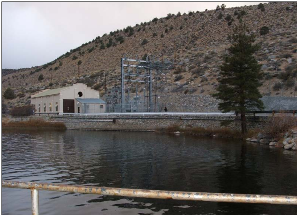
Photo 9.10-8. Plant No. 3/Intake No. 4 Facilities
