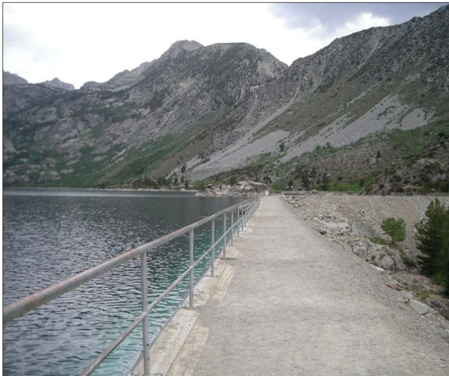
Photo 9.10-20. Lake Sabrina Dam
