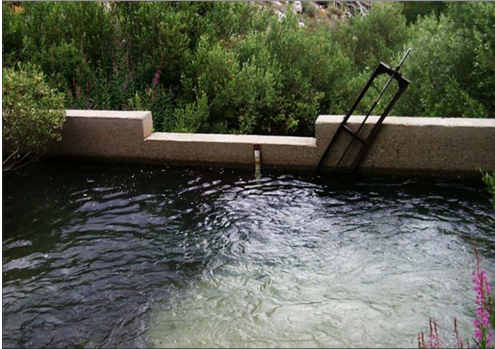
Photo 9.10-15. McGee Creek Diversion
