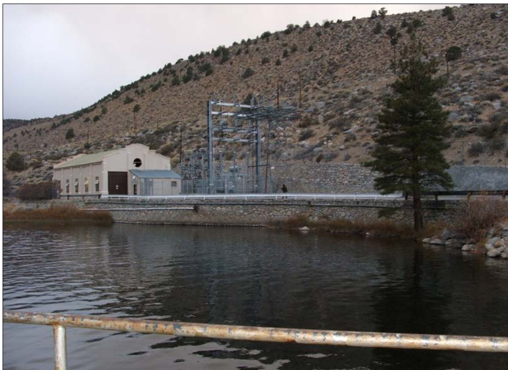
Photo 8.10-8. Plant 3/Intake No. 4 Facilities.
