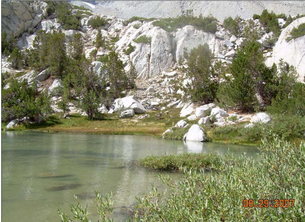
Photo 8.10-17. Below Longley Dam.
