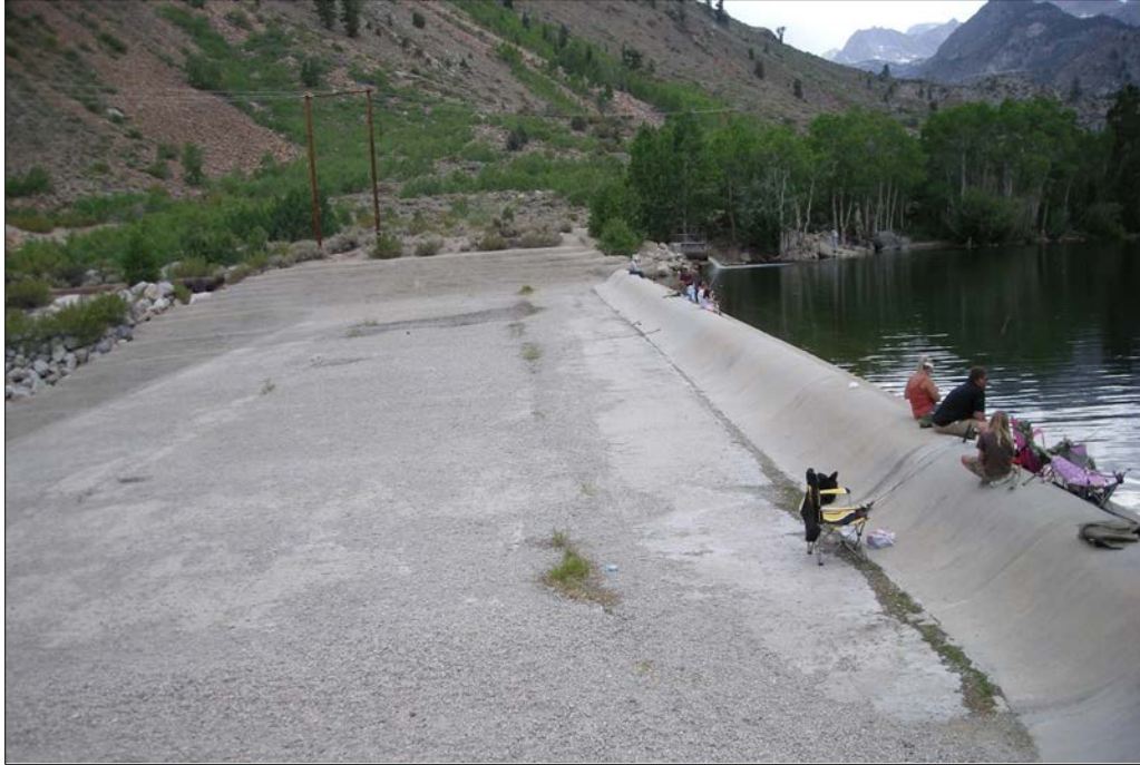
Photo 8.10-13. Intake No. 2 Dam.
