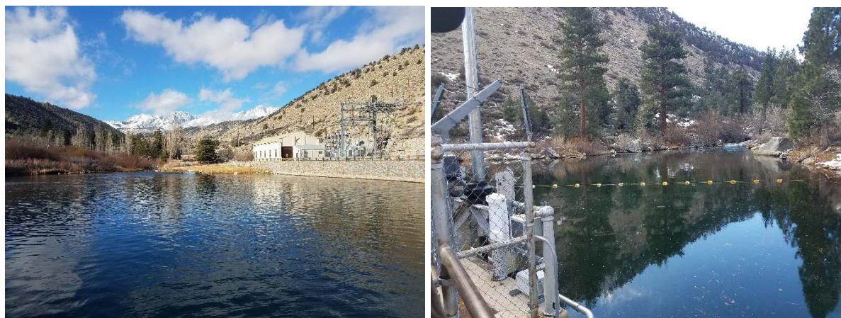
Photo 8.5-2. Plant Intake Forebay Pools.
