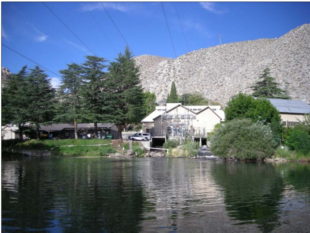
Photo 8.10-6. Plant 4/Intake No. 5.
