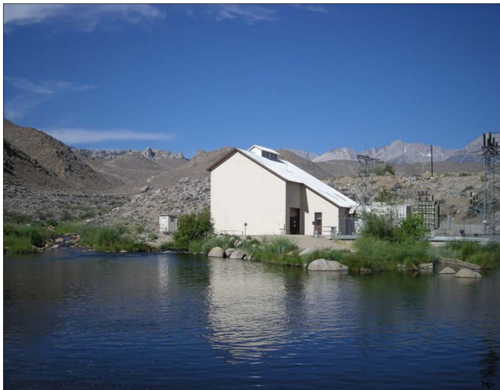
Photo 8.10-4. Plant 5/Intake No. 6.
