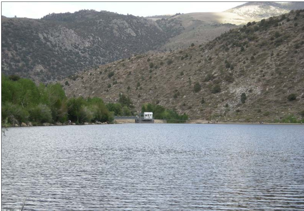
Photo 8.10-12. Intake No. 2 Reservoir and Facilities.
