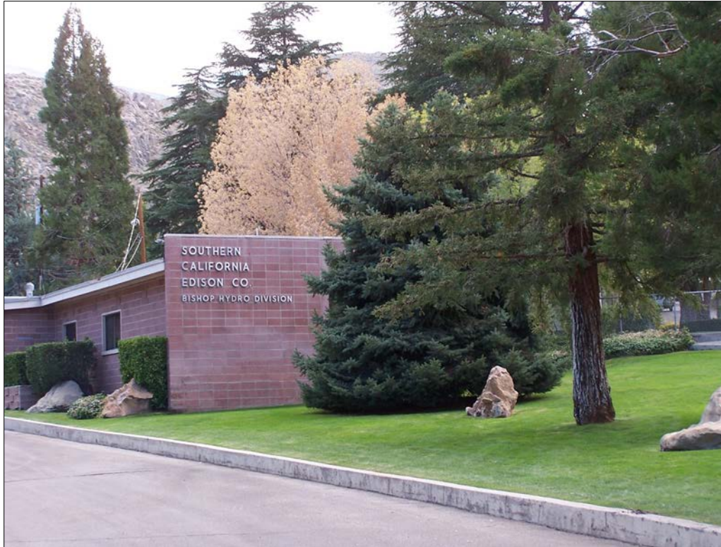
Photo 8.10-7. SCE Office at Plant 4.
