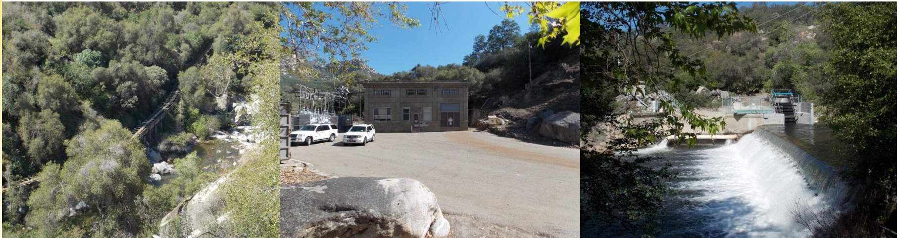
Middle Fork Kaweah River Kaweah No. 3 Flume
