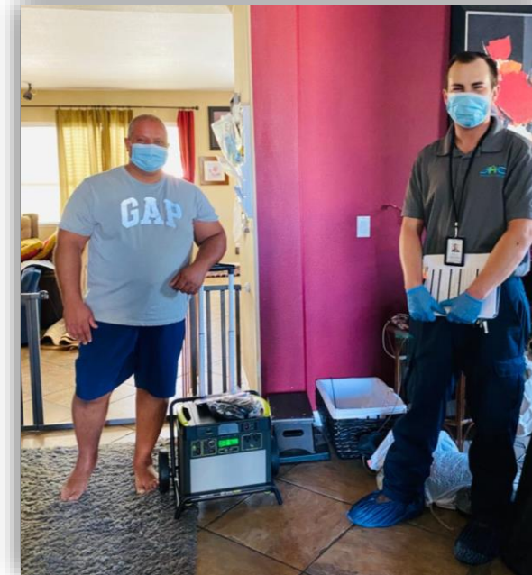
SCE customer with SCE contract representative installing a CCBB
