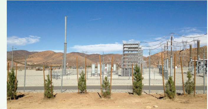
Earlier this year TRTP installed trees around the Vincent Substation.
