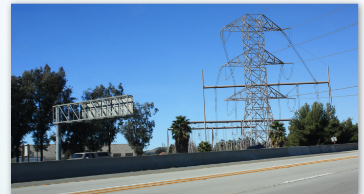
Simulated view looking northwest from State Route 71 toward the ETS.
