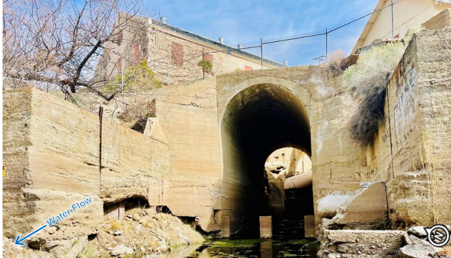
Figure 2-61. Tailrace Outlet at Kern River (Photo Date: 03/2022)
