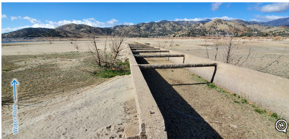
Figure 2-10. Tilley No. 2 Concrete Flume, Looking Downstream (Photo Date: 02/2021)
