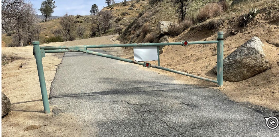
Figure 2-63. Powerhouse Access Road (Photo Date: 03/2022)
