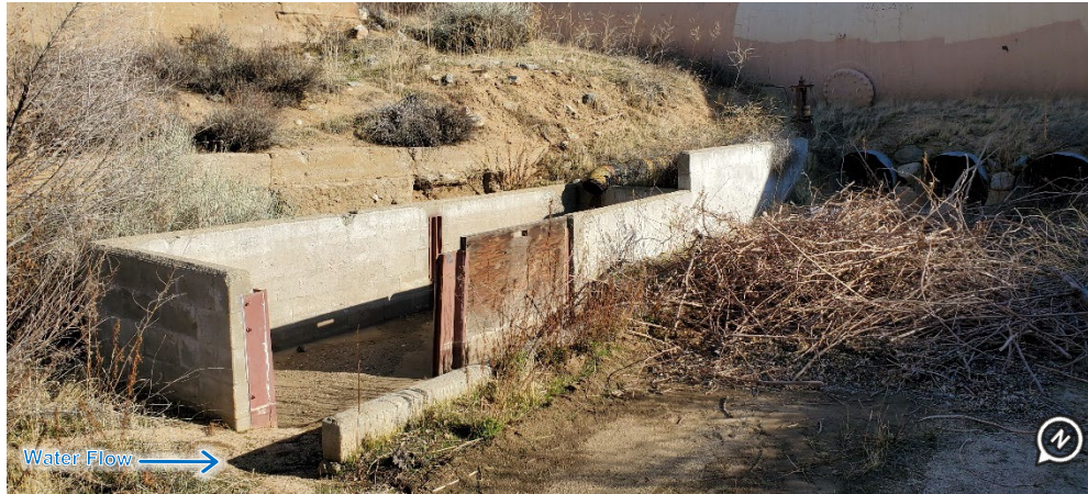
Figure 2-46. Pioneer Steel Siphon Dewatering and Drainage Features (Photo Date: 02/2021)
