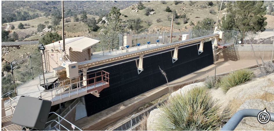
Figure 2-54. Forebay Structure (Photo Date: 02/2021)
