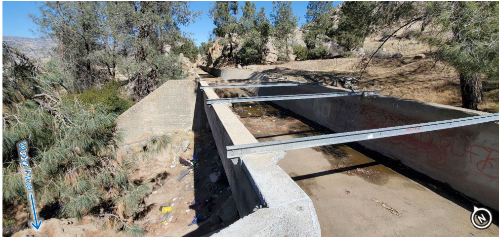
Figure 2-33. School House Cut Flume, Looking Upstream (Photo Date: 02/2021)
