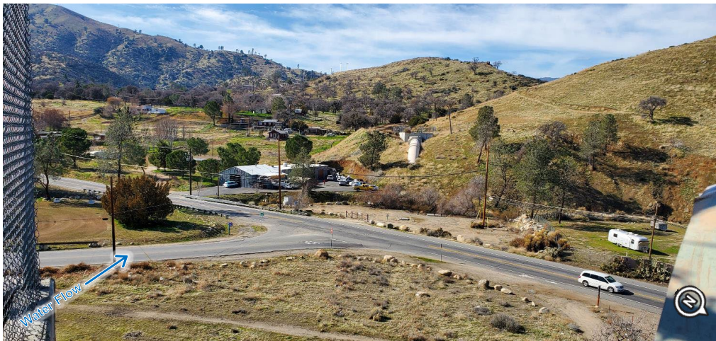
Figure 2-40. Bodfish Siphon, Looking Downstream (Photo Date: 01/2020)
