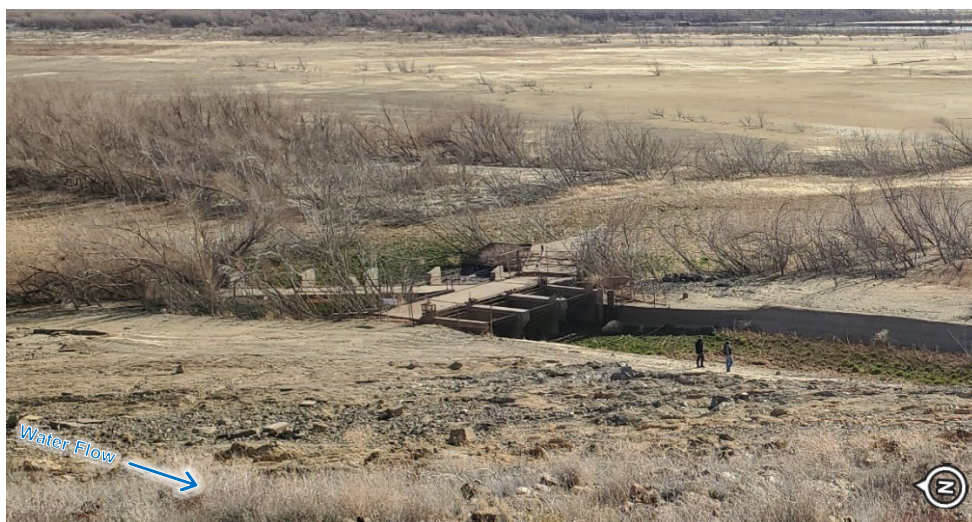
Figure 2-4. Canal Inlet Structures and Concrete-lined Canal, Looking Upstream. (Photo Date: 02/2021)
