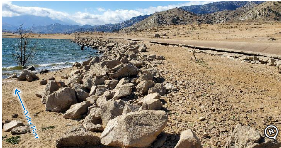
Figure 2-19. Rock Slope Protection on Canal Bank (Photo Date: 02/2021)
