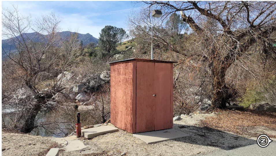
Figure 2-58. Pump House (Photo Date: 03/2022)
