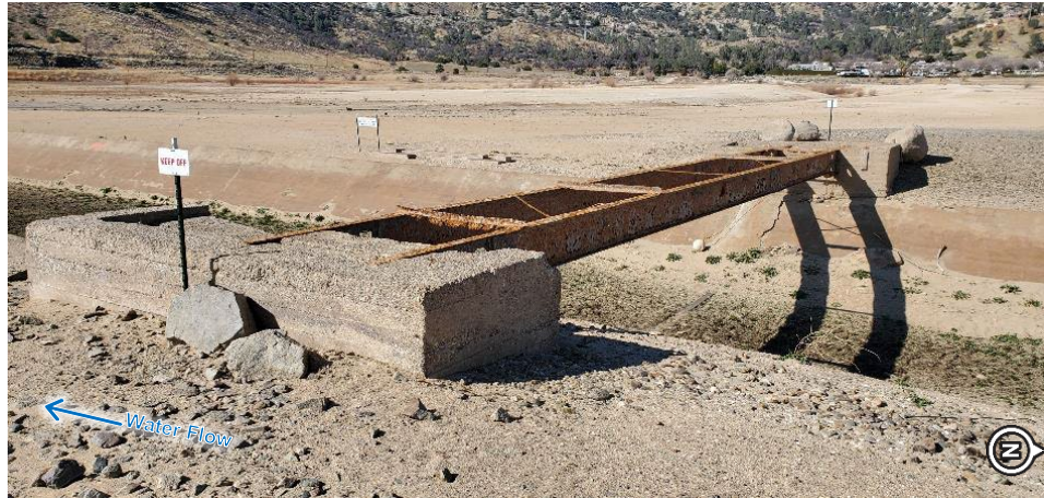
Figure 2-14. Unnamed Steel Bridge near Station 89+00 (Photo Date: 02/2021)
