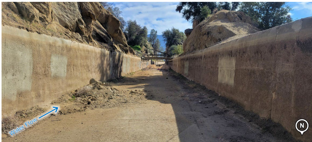
Figure 2-32. School House Cut, Looking Downstream (Photo Date: 03/2022)
