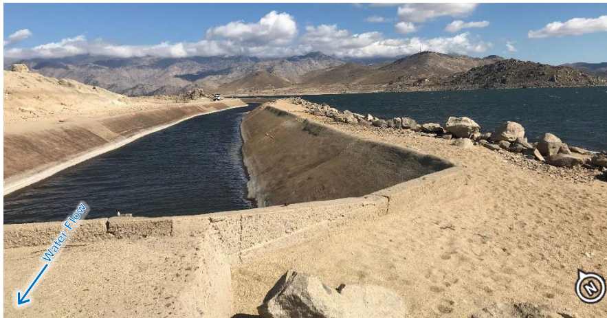
Figure 2-13. Typical Embankment with Rock Slope Protection, Looking Upstream (Photo Date: 02/2021)
