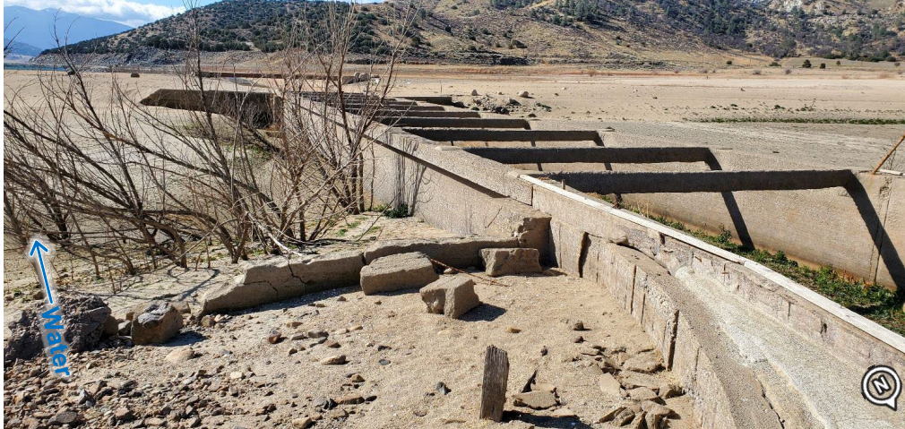
Figure 2-11. Tilley No. 3 Concrete Flume, Looking Downstream (Photo Date: 02/2021)
