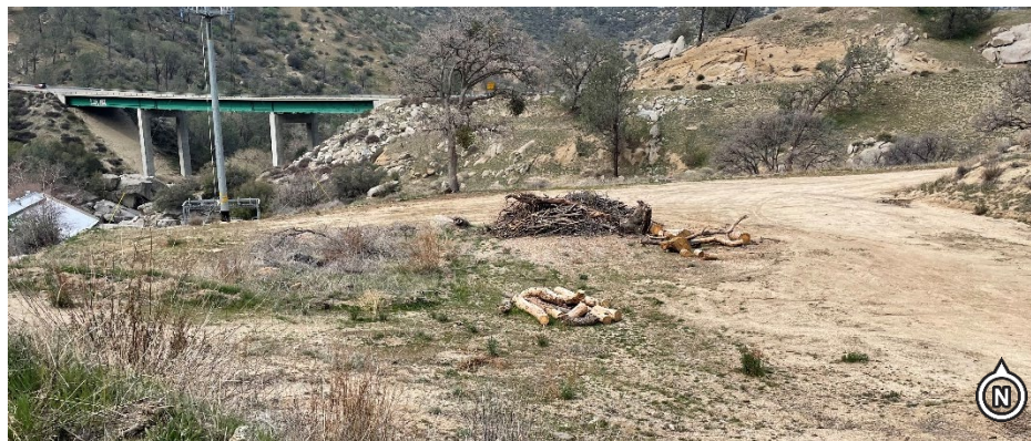
Figure 2-64. Staging Area for Penstock Demolition (Mid-slope) (Photo Date: 03/2022)
