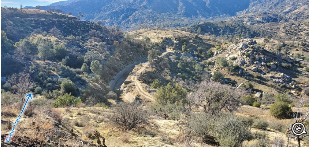
Figure 2-47. Concrete-lined Canal, Looking Downstream of Tunnel No. 1 1/2 (Photo Date: 02/2021)
