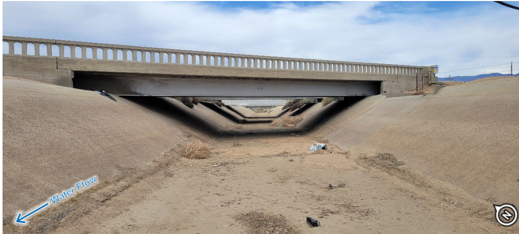
Figure 2-29. Lake Isabella Boulevard Bridge, Looking Upstream (Photo Date: 03/2022)
