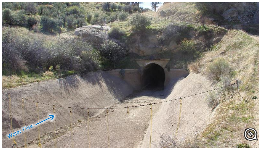
Figure 2-48. Tunnel No. 1 1/2 Entrance, Looking Downstream (Photo Date: 02/2021)
