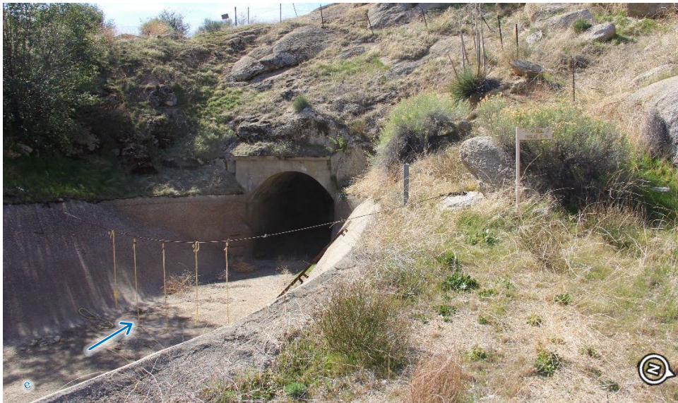
Figure 2-49. Tunnel No. 2 Entrance, Looking Downstream (Photo Date: 02/2021)
