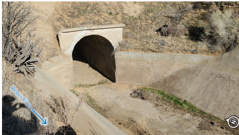
Figure 2-52. Tunnel No. 3 Exit, Looking Upstream (Photo Date: 02/2021)
