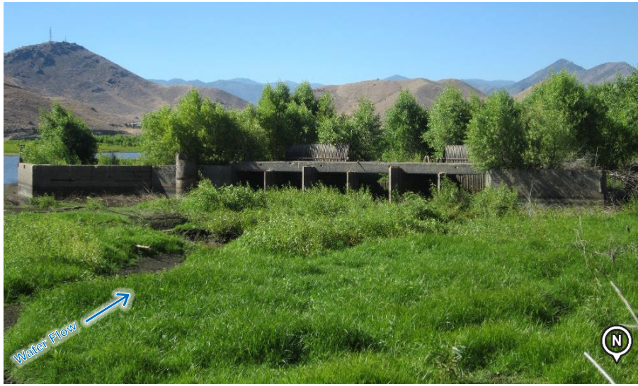
Figure 2-3. Canal Inlet Structure, Looking Downstream (Photo Date: 06/2013)
