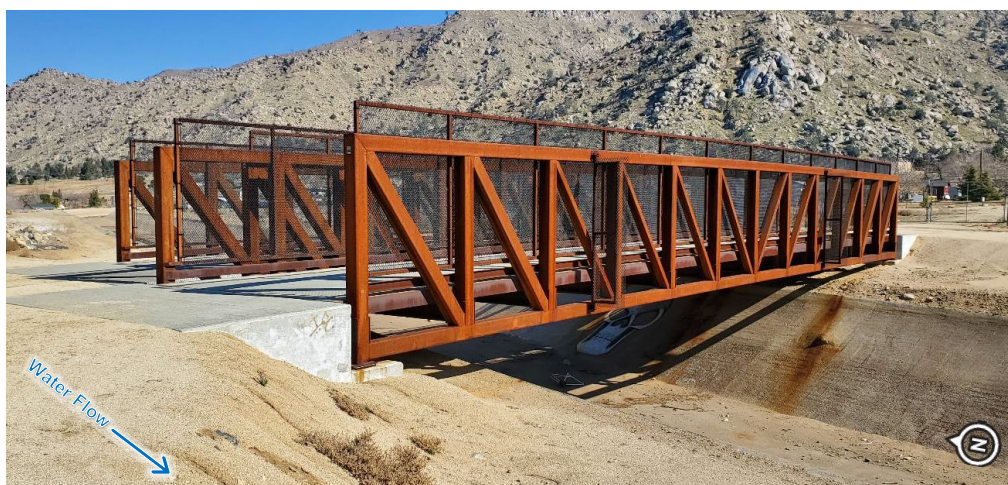
Figure 2-37. County Emergency Vehicular Bridges (Non-Project) (Photo Date: 01/2020)
