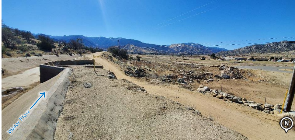
Figure 2-31. School House No. 1 Concrete Flume, Looking Downstream (Photo Date: 02/2021)
