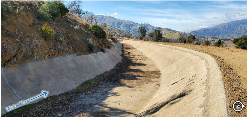
Figure 2-39. Concrete-lined Canal, Looking Downstream (Photo Date: 01/2020)
