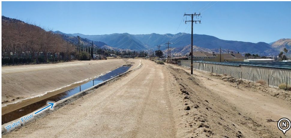
Figure 2-26. Concrete-lined Canal, Looking Downstream (Photo Date: 02/2021)
