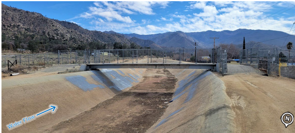
Figure 2-30. Lakeland Walk Bridge (Non-Project), Looking Downstream (Photo Date: 03/2022)
