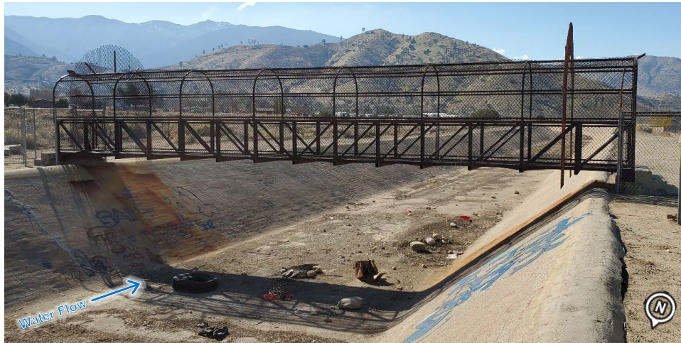
Figure 2-36. School Pedestrian Bridge, Looking Downstream (Photo Date: 01/2020)
