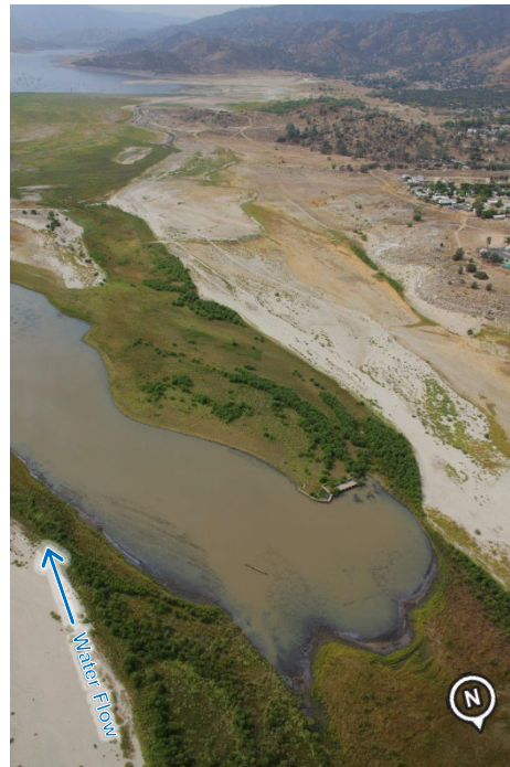
Figure 2-2. Aerial View of the Diversion Dam and Intake Structure, Looking Downstream (Photo Date: 09/2012)
