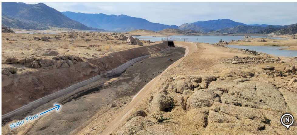
Figure 2-22. Kern River Concrete Siphon Entrance, Looking Downstream (Photo Date: 03/2022)
