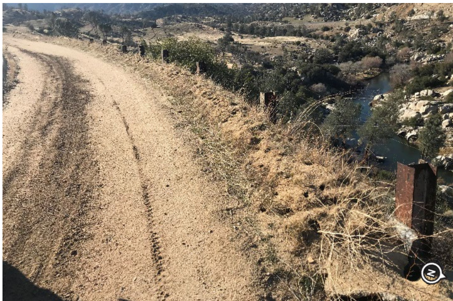
Figure 2-43. Retaining Wall Structure Downstream of Tunnel No. 1, Looking Downstream (Photo Date: 01/2020)
