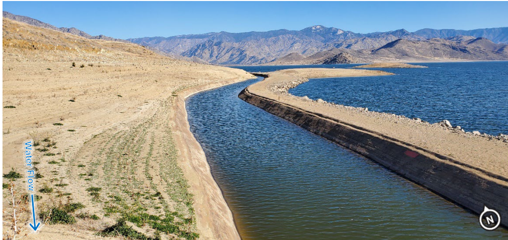
Figure 2-23. Engineers Point, Looking Upstream (Photo Date: 02/2021)
