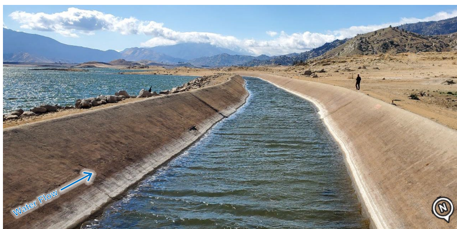
Figure 2-18. Concrete-lined Canal, Looking Downstream (Photo Date: 02/2021)
