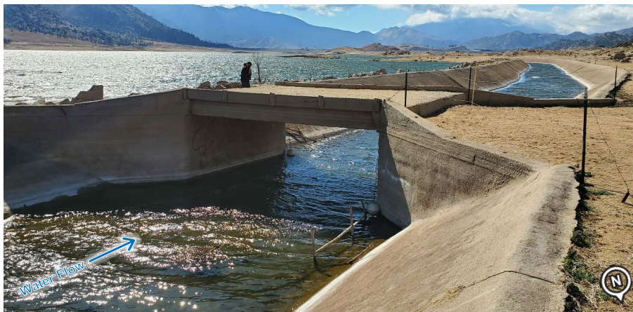
Figure 2-20. Sawmill Bridge at Station 173+50, Looking Downstream (Photo Date: 02/2021)
