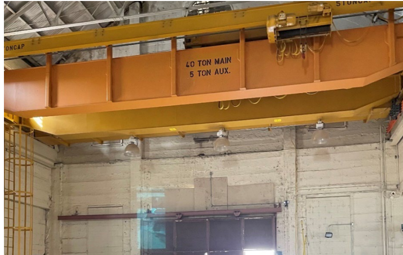
Figure 2-62. Existing Crane (Photo Date: 01/2020)
