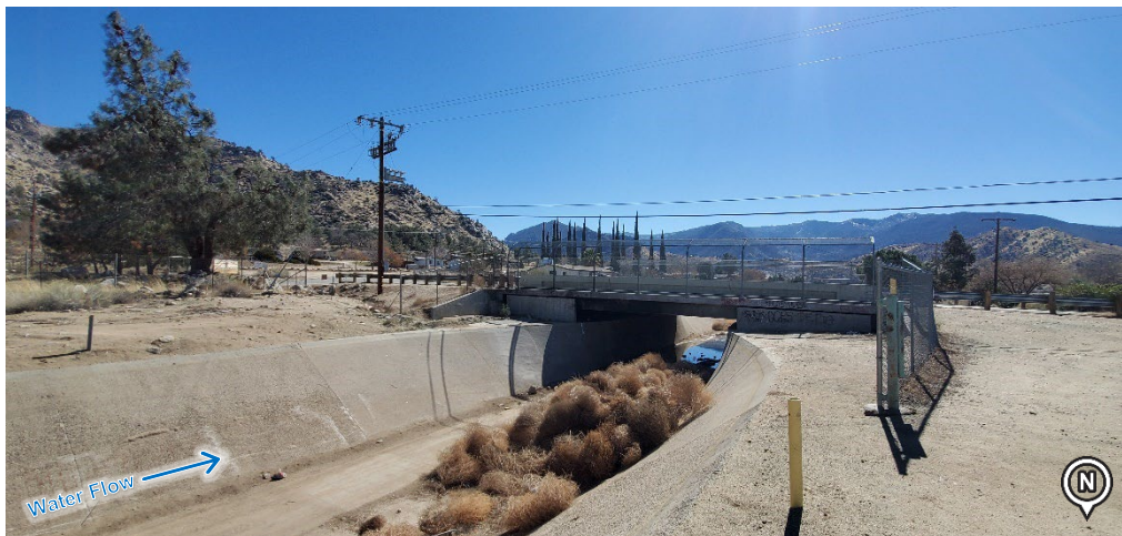
Figure 2-34. Erskine Creek Road Bridge, Looking Downstream (Photo Date: 02/2021)
