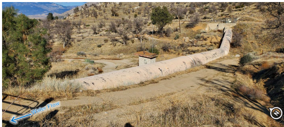
Figure 2-45. Pioneer Steel Siphon, Looking Upstream (Photo Date: 02/2021)
