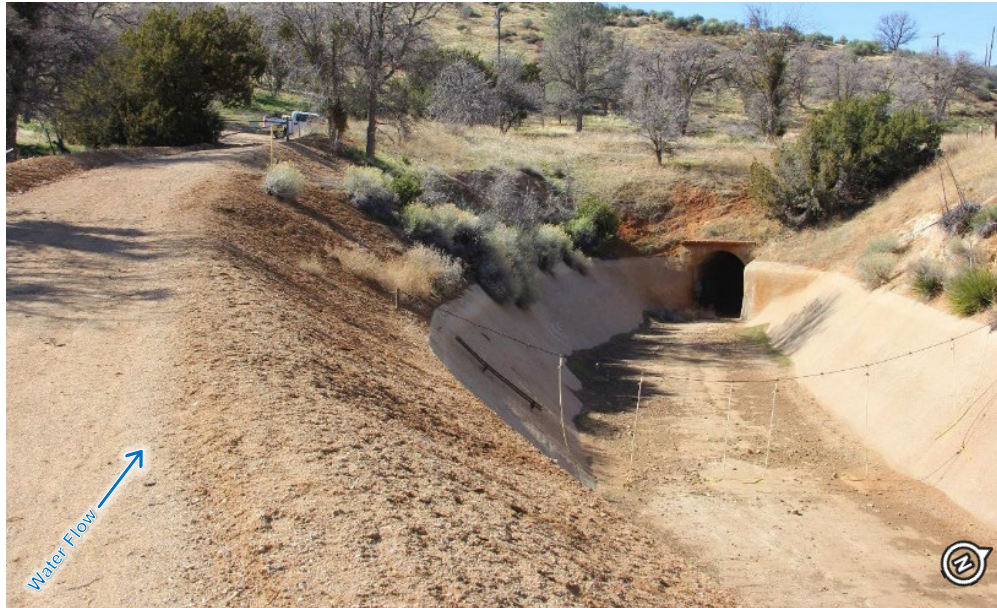
Figure 2-44. Tunnel No. 1 Entrance, Looking Downstream (Photo Date: 06/2020)
