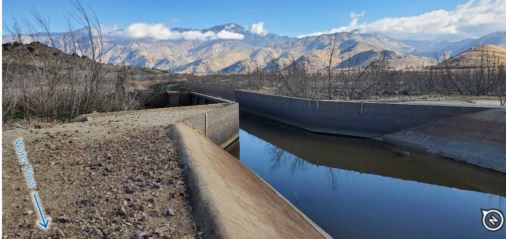
Figure 2-7. Tilley No. 1 Concrete Flume, Looking Upstream (Photo Date: 02/2021)
