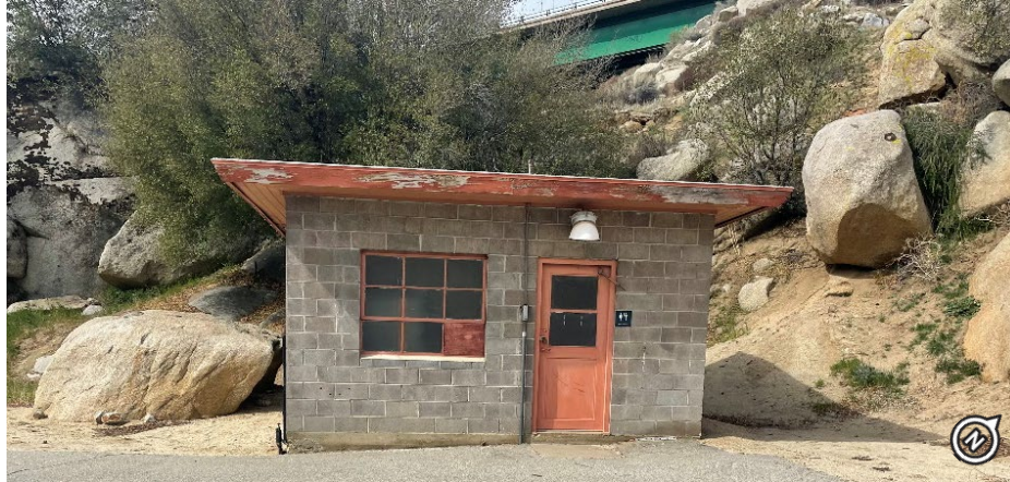
Figure 2-59. Restroom/Outbuilding at Powerhouse (Photo Date: 03/2022)
