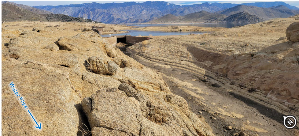
Figure 2-21. Rich Gulch Concrete Siphon Exit, Looking Upstream (Photo Date: 03/2022)
