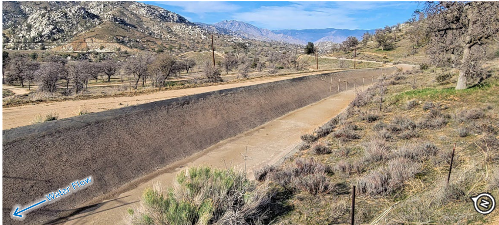
Figure 2-42. Concrete-lined Canal, Looking Upstream (Photo Date: 03/2022)
