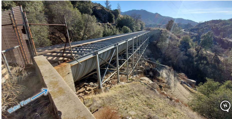
Figure 2-53. Profanity Steel Flume, Looking Downstream (Photo Date: 02/2021)
