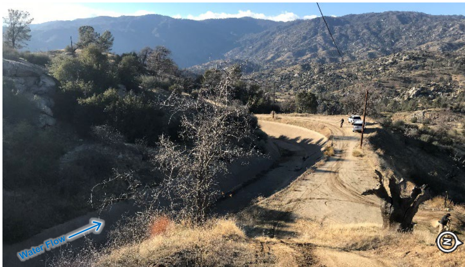
Figure 2-50. Utility Poles on Right Bank Downstream of Tunnel No. 2, Looking Downstream (Photo Date: 02/2021)
