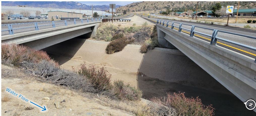
Figure 2-28. SR 178 Bridges (Photo Date: 03/2022)
