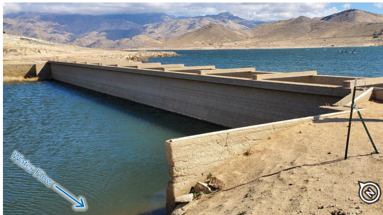
Figure 2-15. Refugio Concrete Box Flume (near Station 149+00), Looking Upstream (Photo Date: 02/2021)
