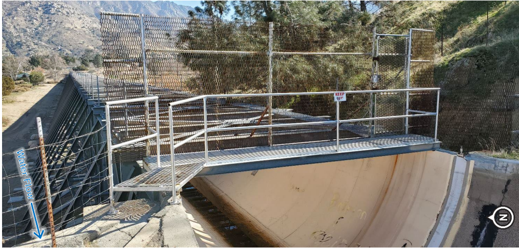
Figure 2-38. Erskine Creek Flume, Looking Upstream (Photo Date: 01/2020)
