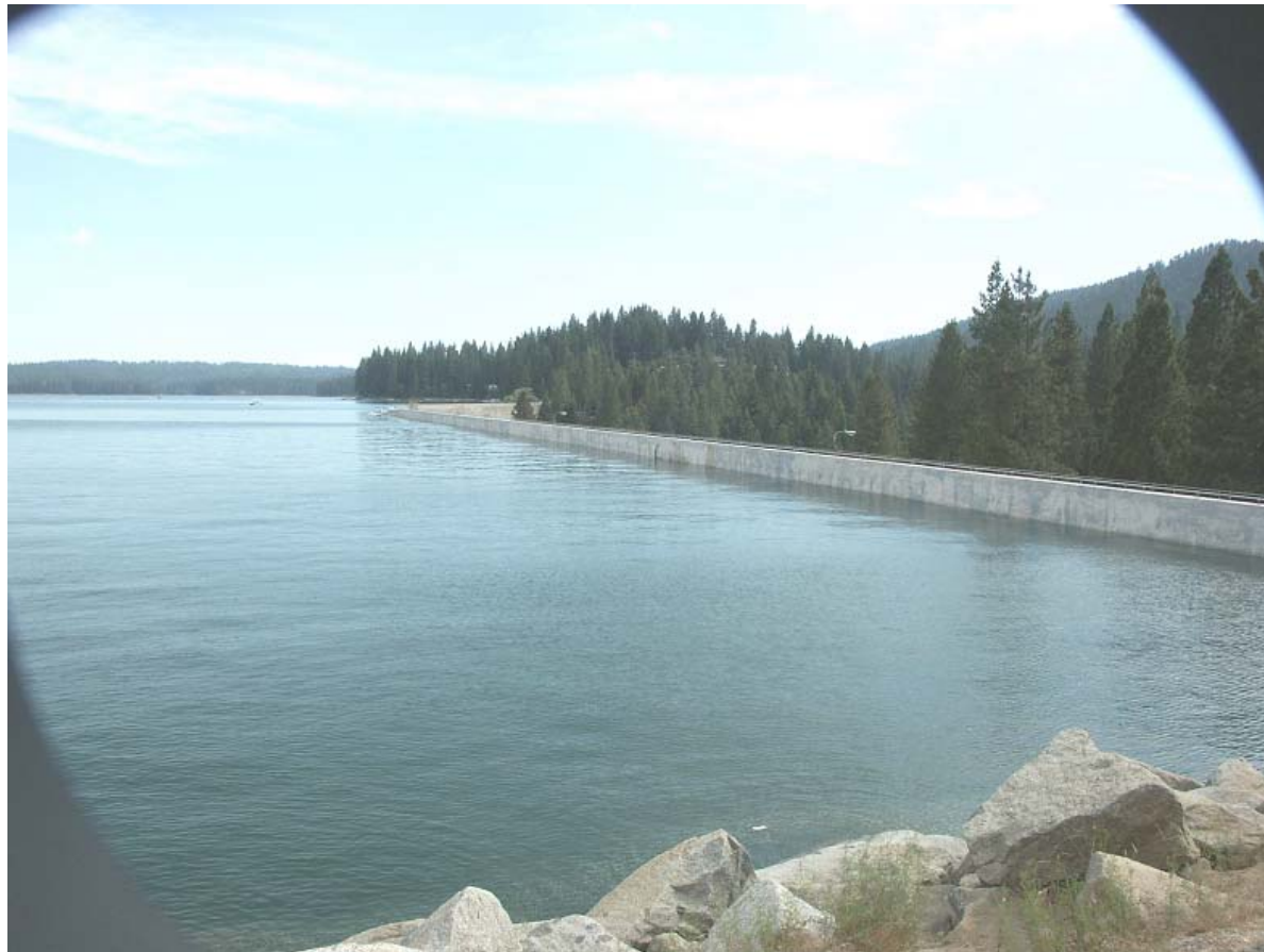
Shaver Lake and Dam View South from Shaver Dam Turnout Water Surface Elevation at 5,365 feet
