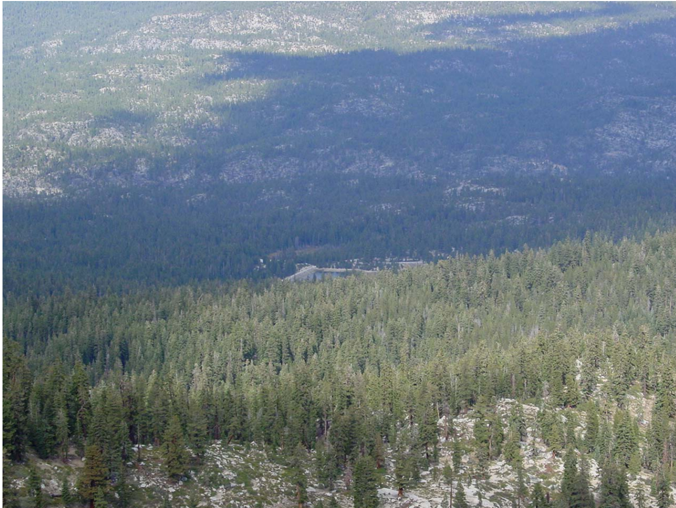
KOP 10 - Photo 10c View of Portal Forebay looking east from White Bark Vista (October 1, 2001)
