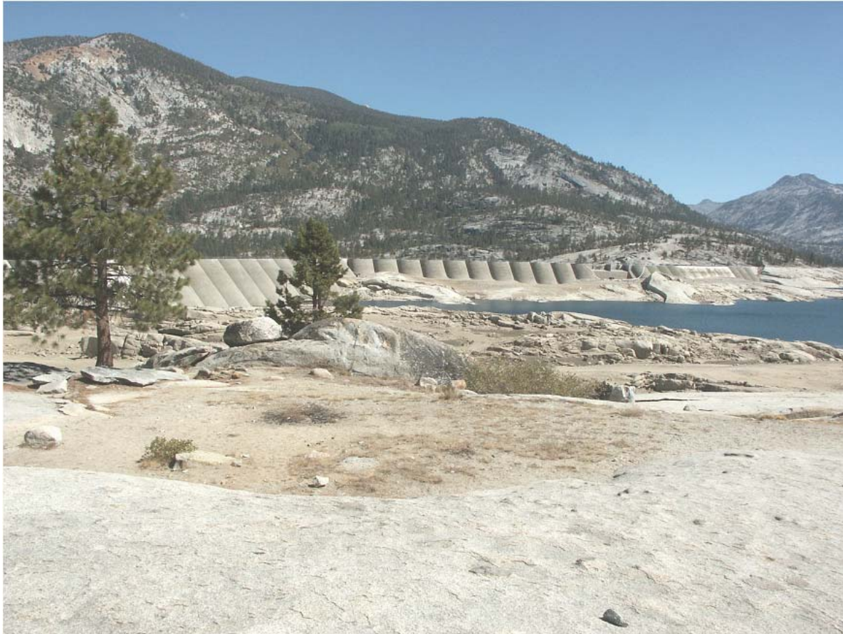
Florence Lake Boat Launch Water Surface Elevation at 7,261 feet
