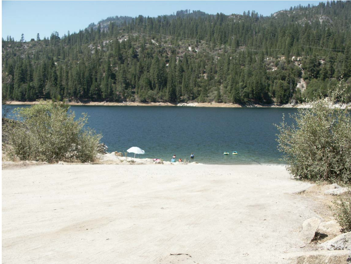
Mammoth Pool Boat Launch View South of Mammoth Pool Boat Ramp Water Surface Elevation at 3,315 feet
