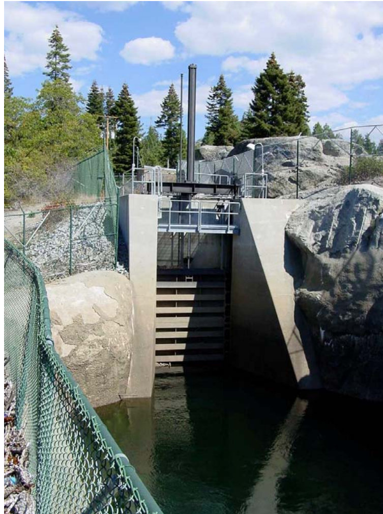
KOP 19 - Photo 19b View of Balsam Meadows inlet looking north east from Balsam Meadows Forebay (October 2, 2001)
