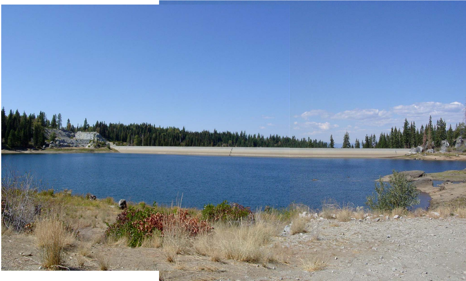
KOP 19 - Photo 19a View of Balsam Meadows Forebay and Dam looking north east from Balsam Meadows Forebay Day Use Area (October 2, 2001)
