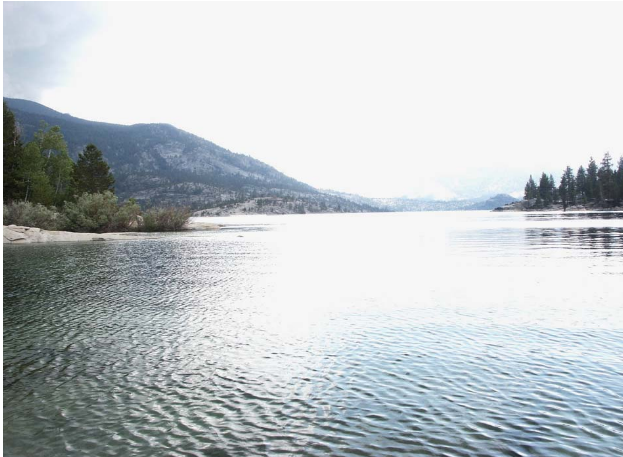
KOP 11 - Photo 11 View of Florence Lake Dam looking east from Florence Lake Picnic Area (July 2, 2002)
