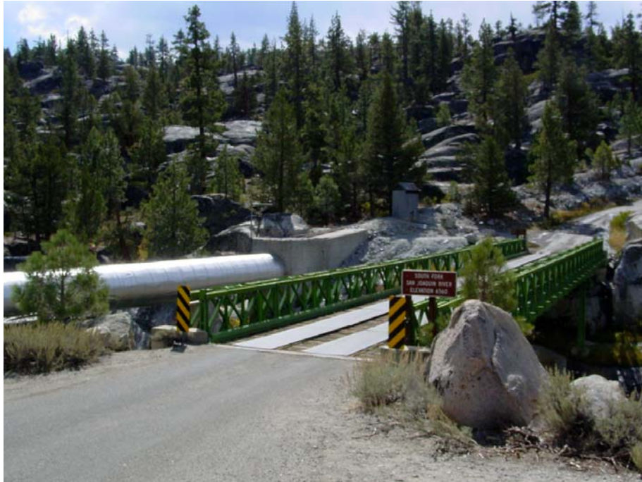
KOP13 - Photos 13a View of Mono Bear Siphon looking south from Kaiser Pass Road (October 1, 2001)
