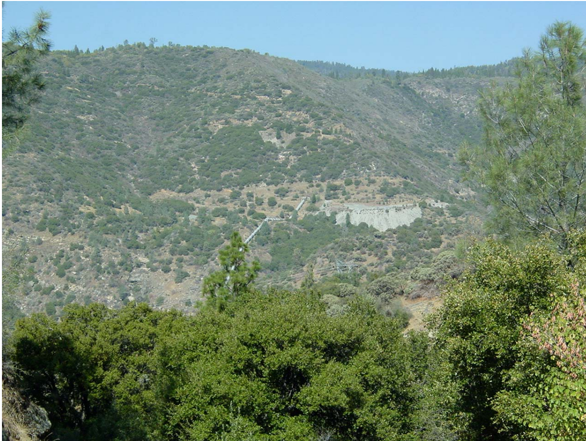
KOP 31 - Photo 31 View of Mammoth Pool penstock north west from Canyon Road between Big Creek No. 2/2A and Big Creek No. 8 (October 4, 2001)
