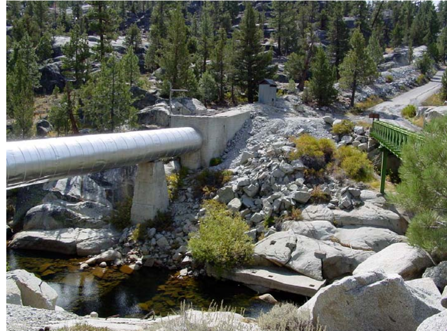
KOP13 - Photos 13b View of Mono Bear Siphon looking south from Kaiser Pass Road (October 1, 2001)
