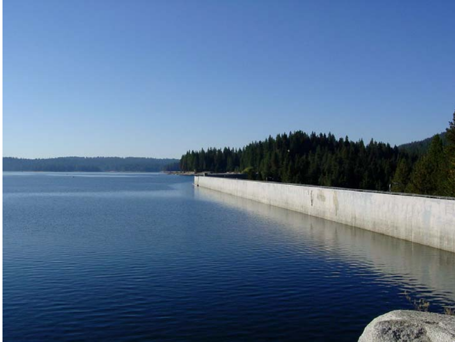
KOP 15 - Photo 15a View of Shaver Lake Dam looking south from Shaver dam turnout (October 3, 2001)
