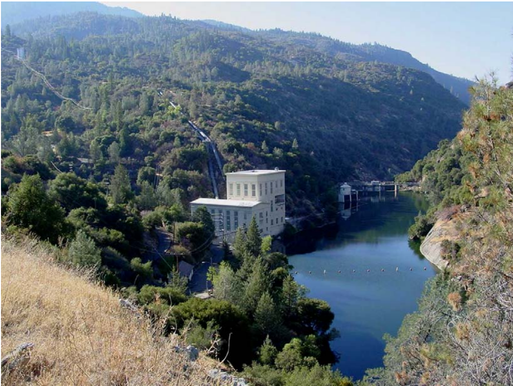
Photo C-13 - Powerhouse No. 8. Powerhouse No. 8 and the associated facilities are located at the confluence of Big Creek and the San Joaquin River in a steep walled canyon at an approximate elevation of 2,200 feet. This location is within a vegetation community consisting of chaparral and oak woodland.
