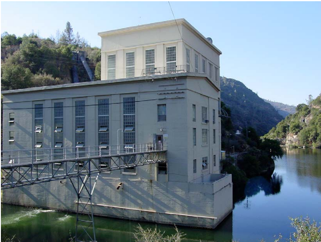
Photo C-14 – Powerhouse No. 8. This photograph shows the powerhouse surrounded along three sides by the Dam 6 forebay and therefore has a low fire risk or hazard.
