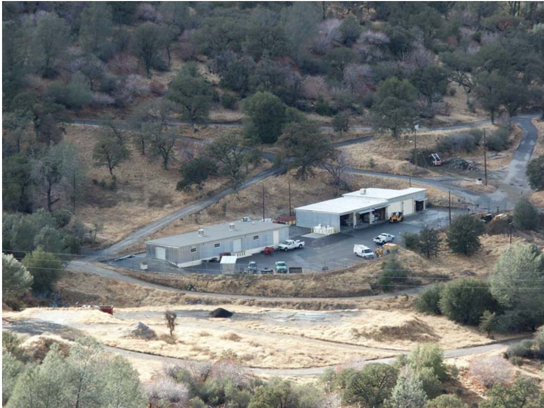
Photo C-19 – Big Creek No. 3 Community. This photograph shows the workyard/corporation yard in the Big Creek No. 3 community and depicts the defensible clearing of brush from open areas and around the perimeter of the facility. Ground fuels in the oak woodland setting consists predominately of grass and leaves.
