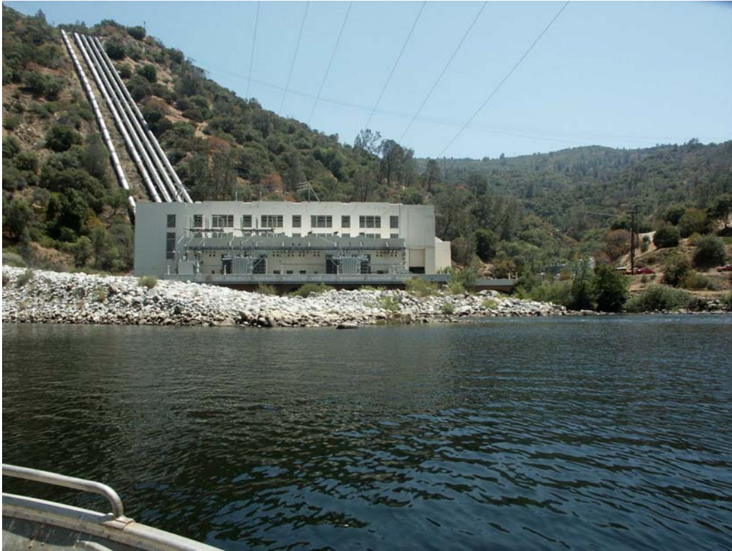
Photo C-20 – Powerhouse No. 3. This photograph shows the powerhouse located at the base of a steep canyon with the hillside above the powerhouse building covered with thick brush.
