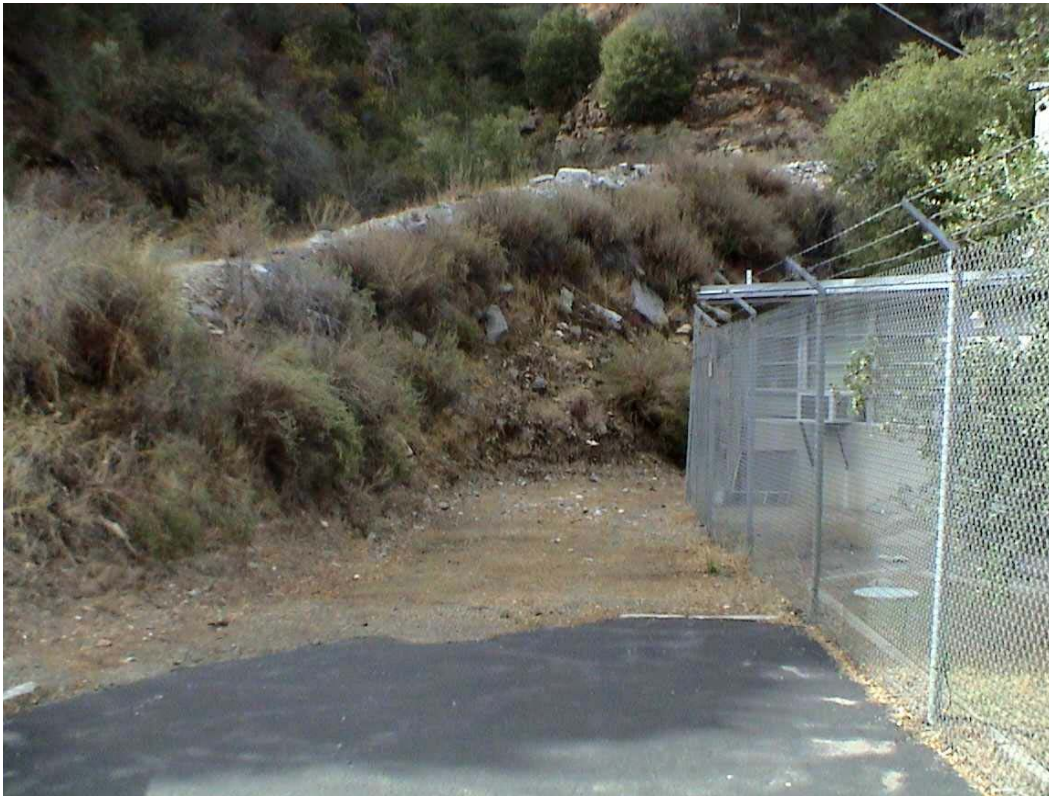
Photo C-17 – Mammoth Pool Powerhouse. This photograph shows the defensible space cleared of brush, grass and woody debris that is maintained around the perimeter of the Mammoth Pool Powerhouse.
