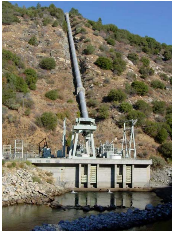
Photo C-16 - Mammoth Pool Powerhouse. This photograph shows the powerhouse located along the San Joaquin River in a steep walled canyon at an approximate elevation of 2,200 feet. This location is within a vegetation community consisting of chaparral and oak woodland.
