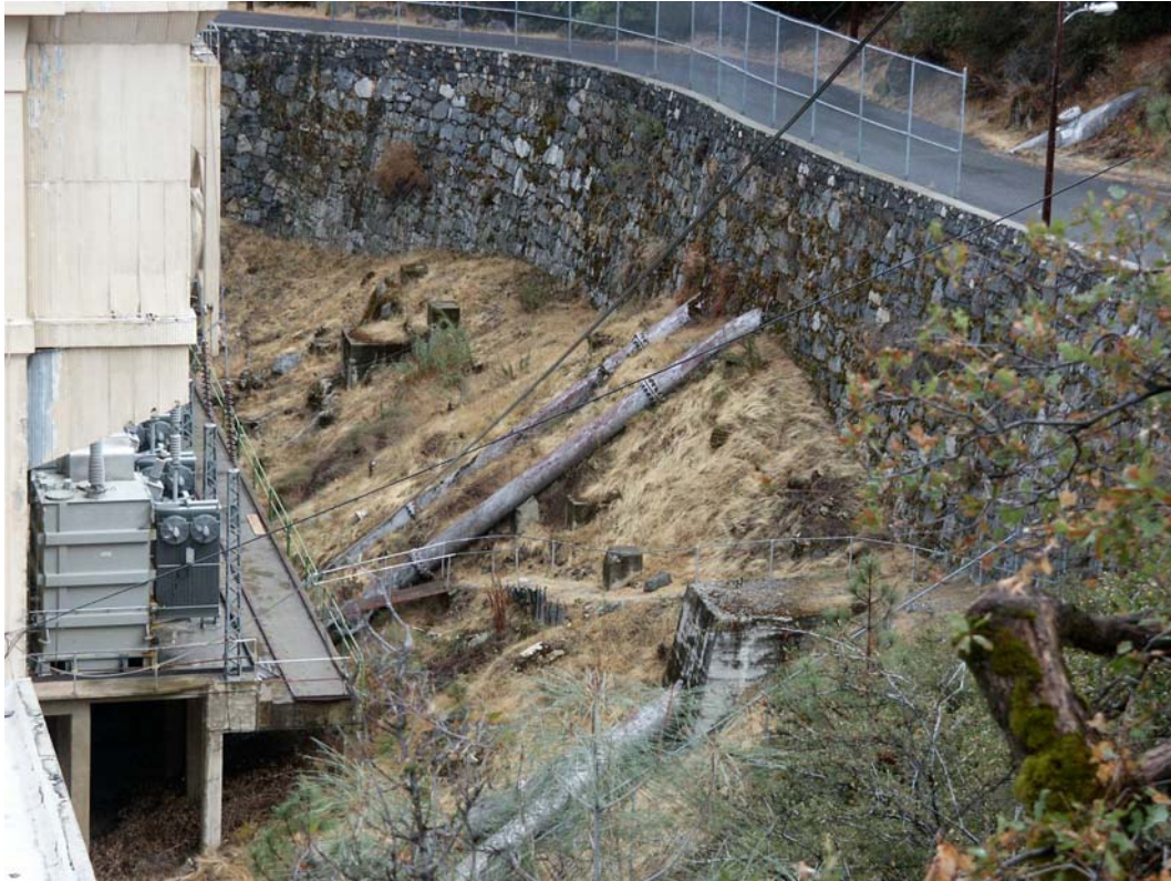
Photo C-10 – Powerhouse 2/2A. This photograph depicts the area immediately behind Powerhouse No. 2/2A. The road, rock wall and perimeter area that is clear of woody debris and brush provides defensible space. The building is of concrete wall construction which provides good fire protection.
